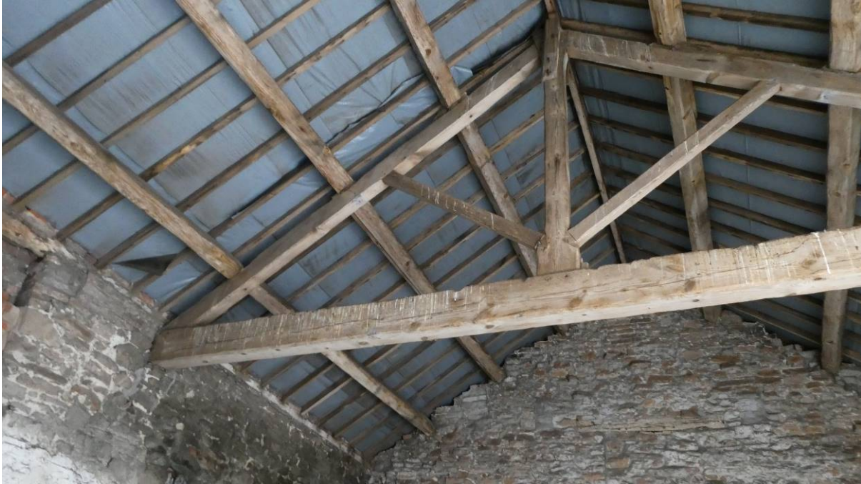
Above: Stone Barn internal view showing original principal roof timbers to be retained
