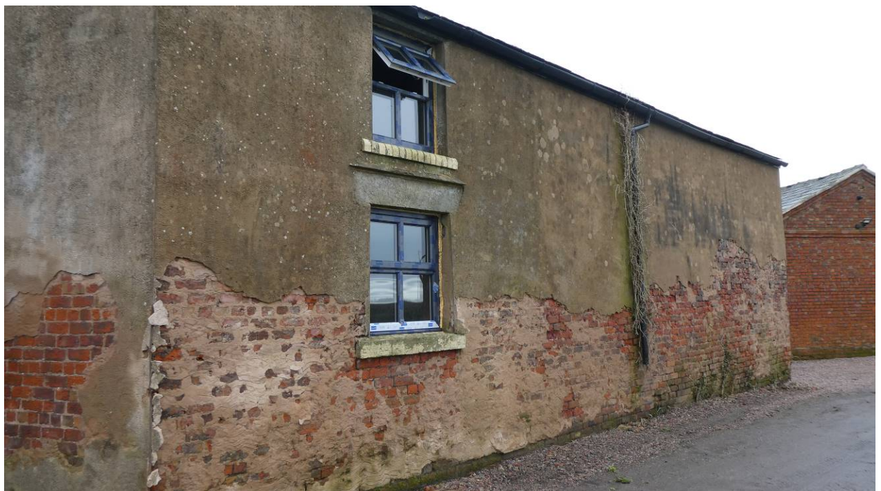
Above: Stone Barn annexe north west external elevation
