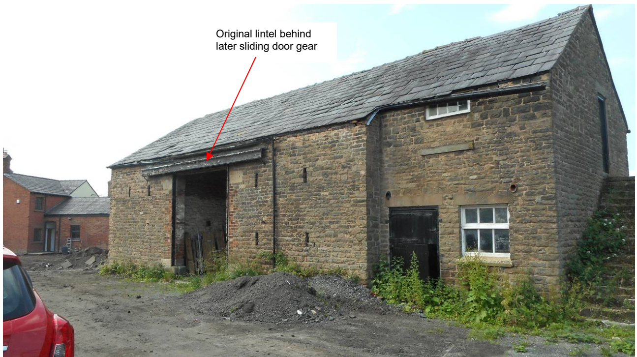
Above: Stone Barn east facing elevation
