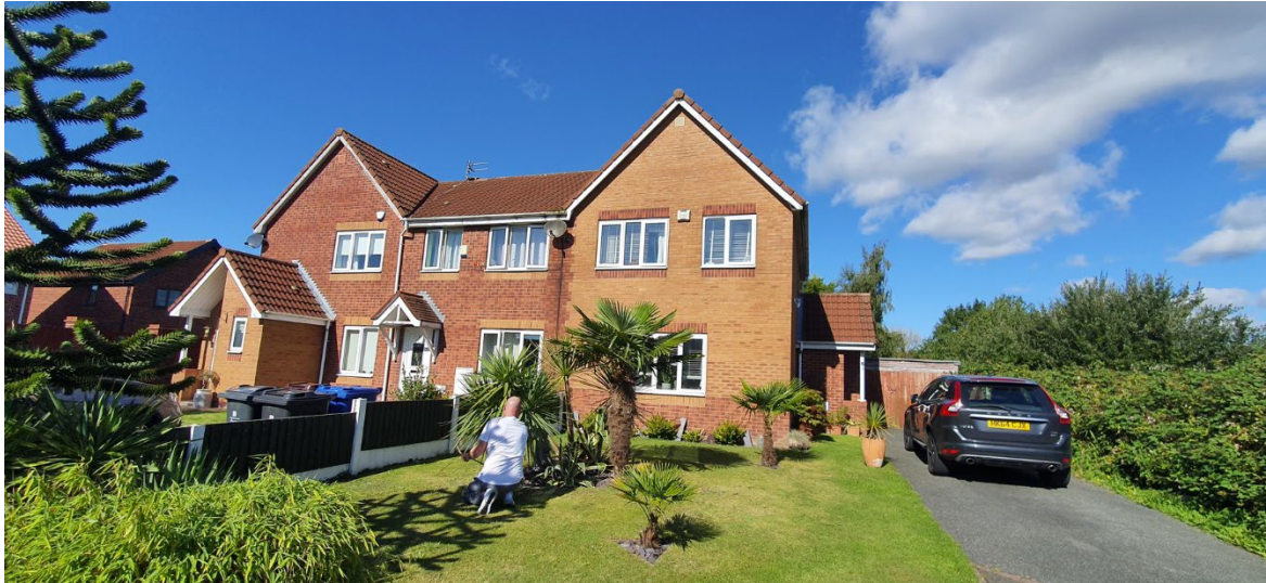
Photograph of the front elevation (looking North West). Existing porch to the right.
