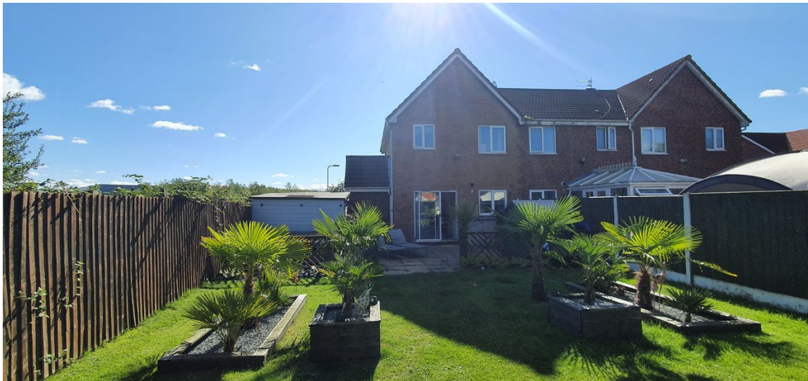
Photograph of the rear elevation (looking South East).
