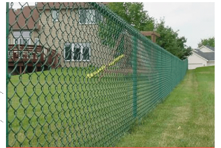
2000 high perimeter chain link fencing to be PPC coated (RAL 9005 - Green) with 60x60 posts at 2000 ctrs.
