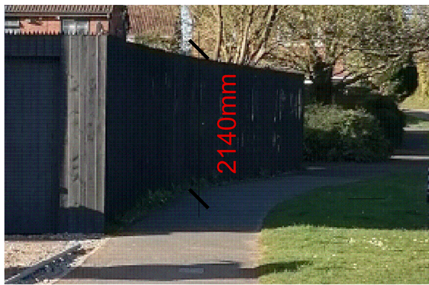
New Fence line Adjacent Manorwood Drive
