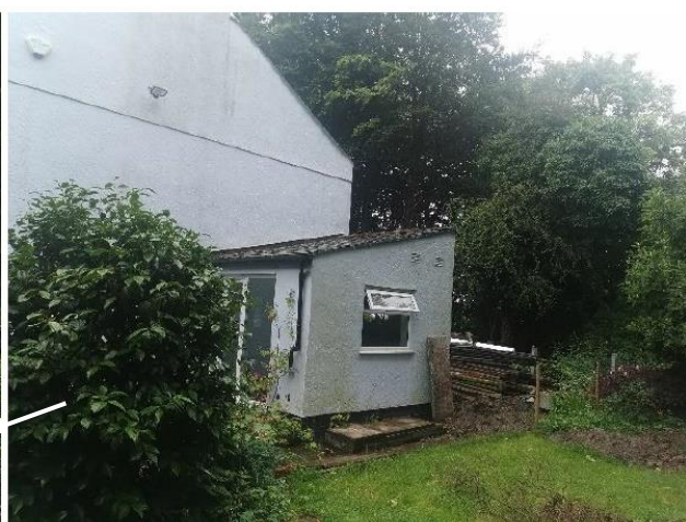
North / east of rear extension.
