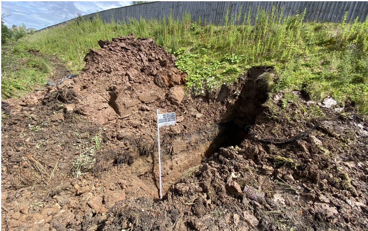
Photograph 18 – TT09 excavated to 4.4m bgl. Trial Trench dug into the noise bund to locate SHAFT346391-016.
