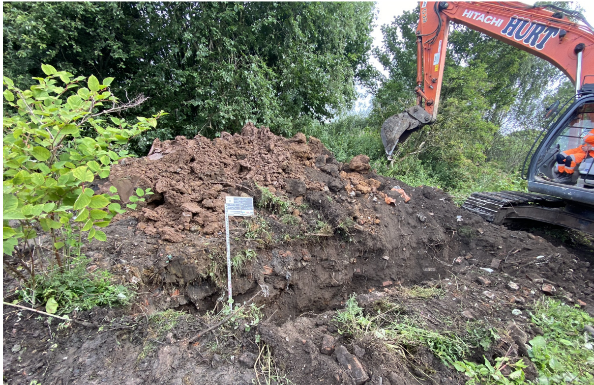
Photograph 17 – TT04 excavated to 4.3m bgl.
