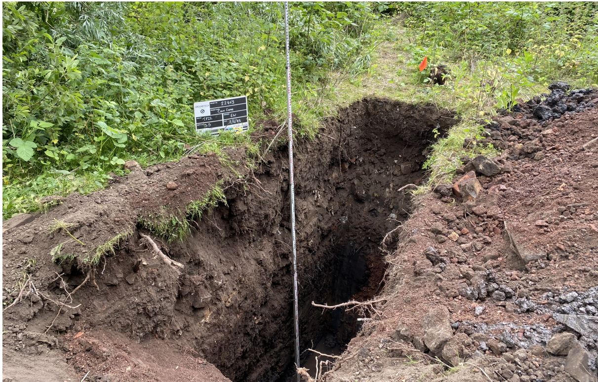
Photograph 13 – TP22 excavated to 3.5m bgl.
