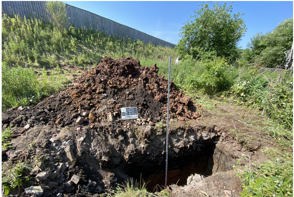
Photograph 12 – TP08 excavated to 3.5m bgl. No evidence of mine entry.
