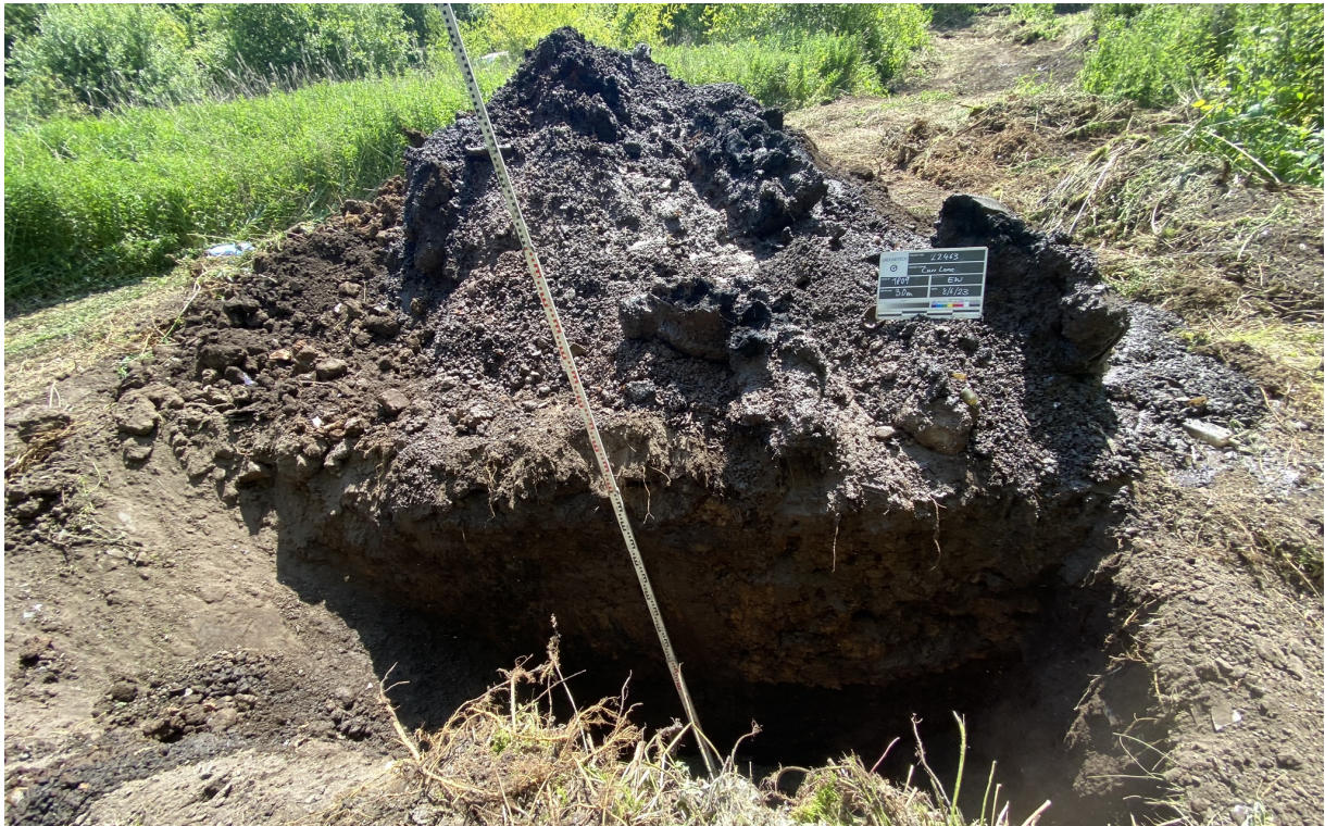
Photograph 11 – TP09 excavated to 3.0m bgl. No evidence of quarry high wall.
