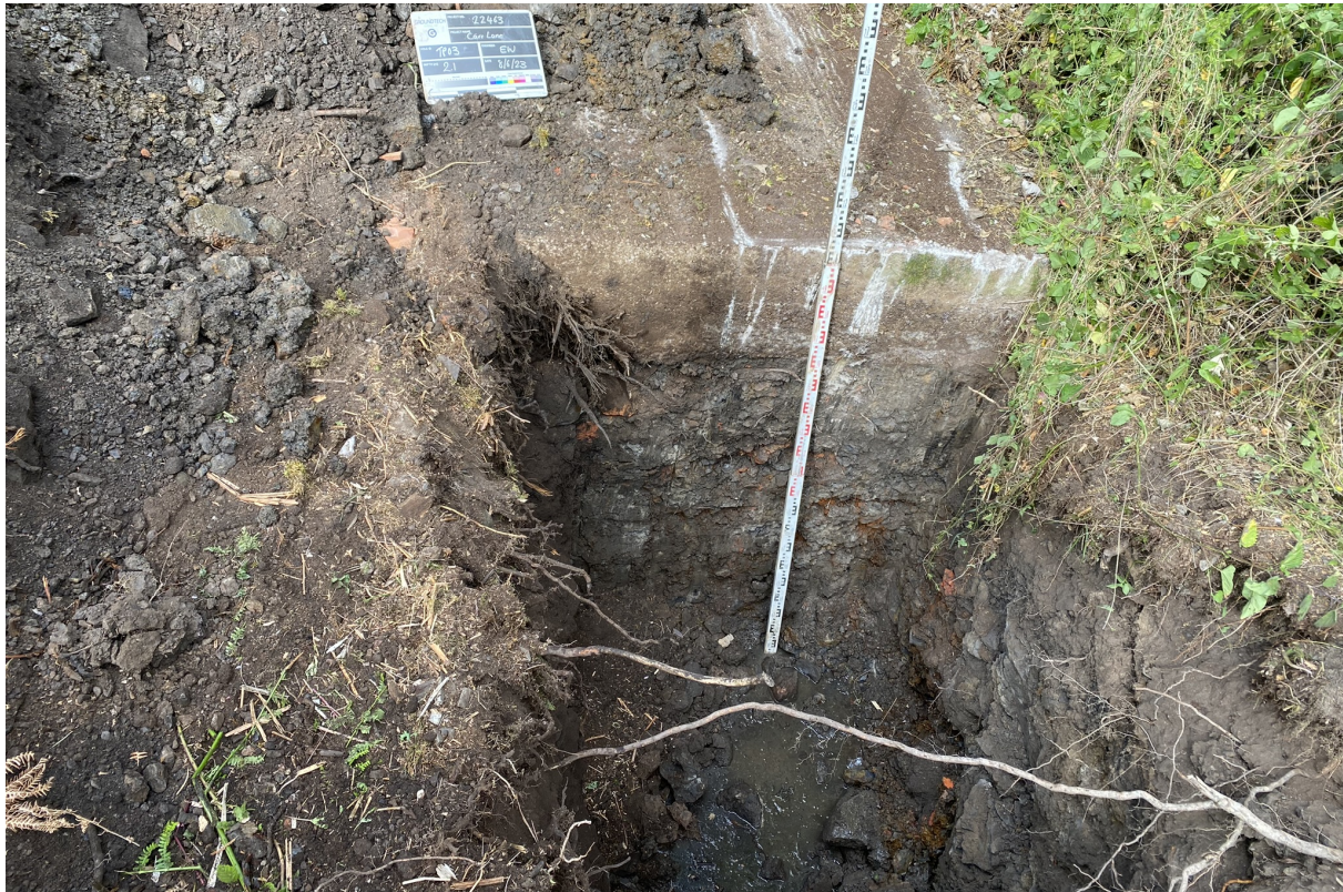
Photograph 9 – TP03 excavated to 2.1m bgl depicting the thickness of the capped mine shaft entry in the south of the site.
