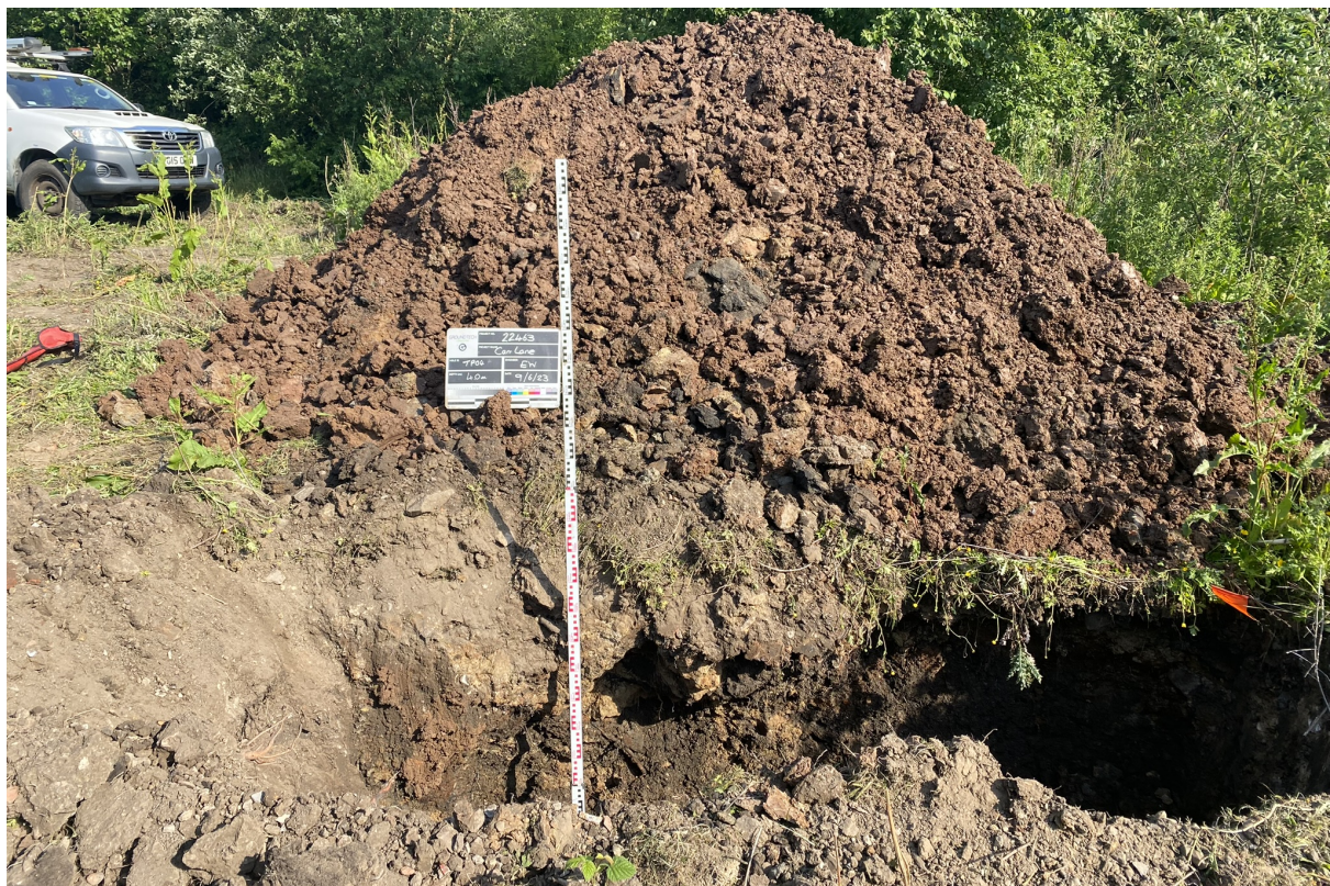
Photograph 10 – TP04 excavated to 4.0m bgl. No evidence of mine entry.
