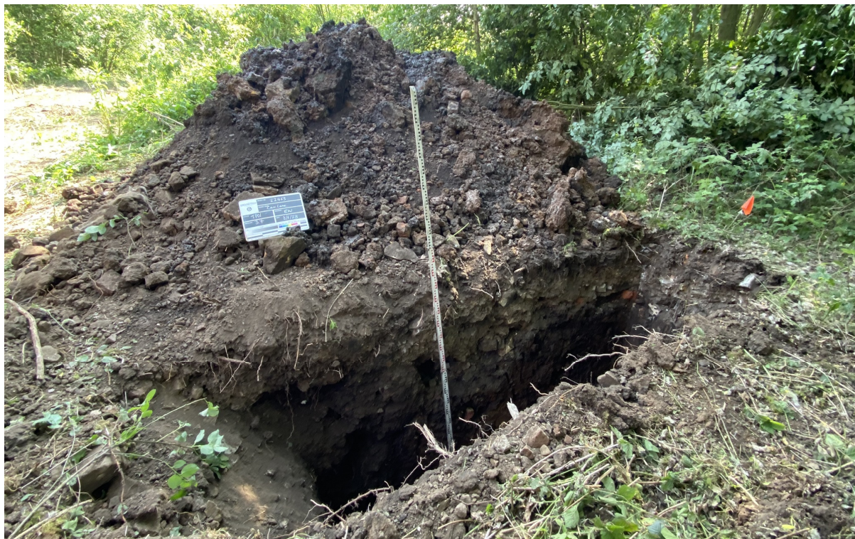
Photograph 7 – TP01 excavated to 3.7m bgl.
