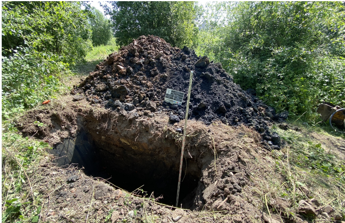
Photograph 8 – TP02 excavated to 4.0m bgl. The colliery spoil is visible in the right of the spoil heap.
