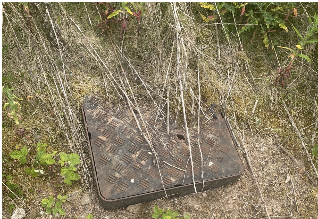
Photograph 4 – Water utility cover along the eastern boundary.
