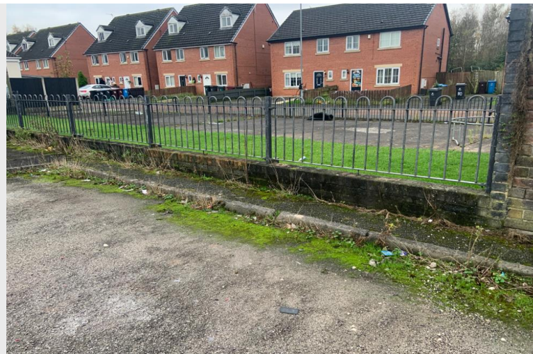
Photograph 6: View of the surrounding metal fence
