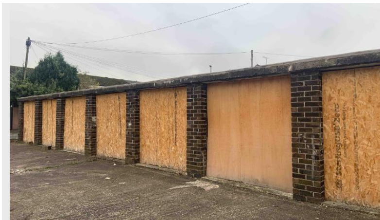
Photograph 1: Abandoned seven-unit garage building
