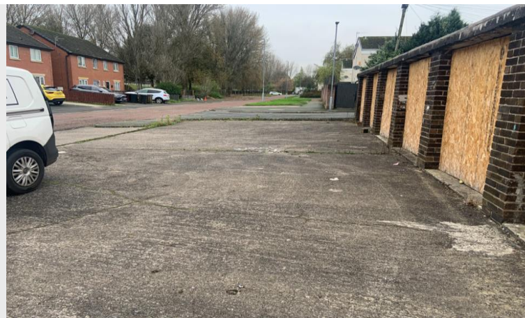
Photograph 2: Area of hardstanding to the front of the garage building
