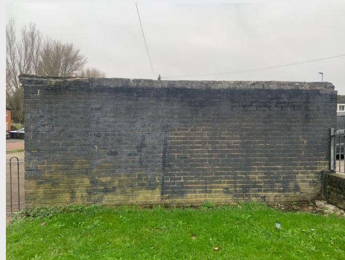
Photograph 8: View of the southeastern side of the building.
