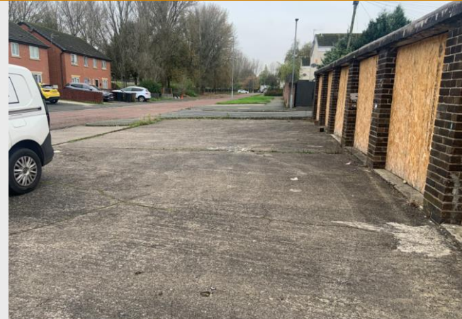
Photograph 2: View of the front of the garage with predominantly hardstanding.
