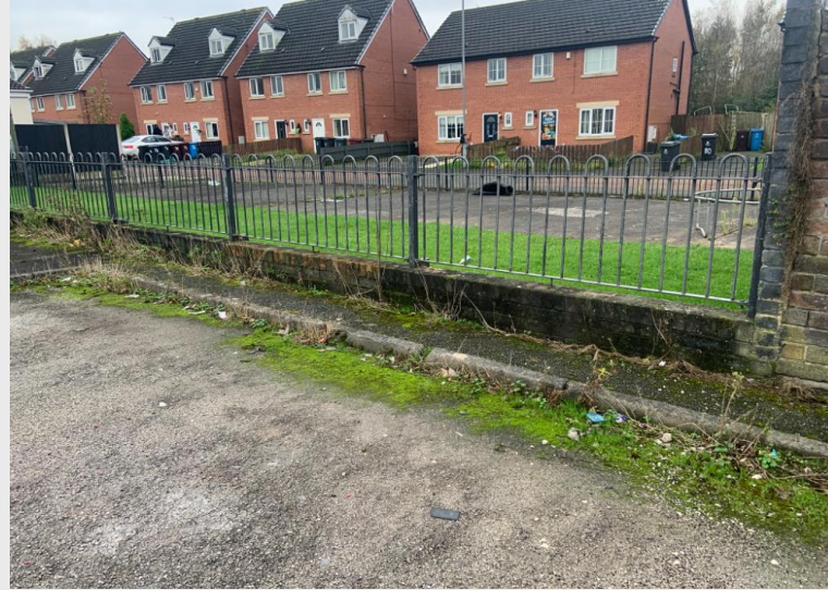
Photograph 5: View of the surrounding metal fencing.
