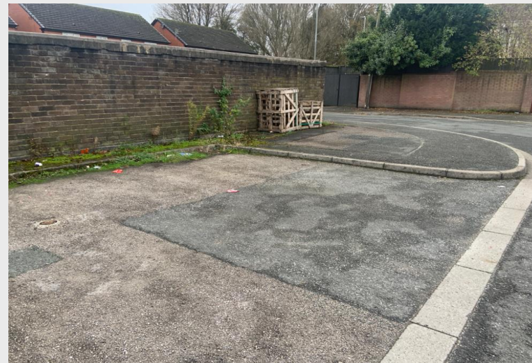
Photograph 4: Hardstanding ground behind the unit.
