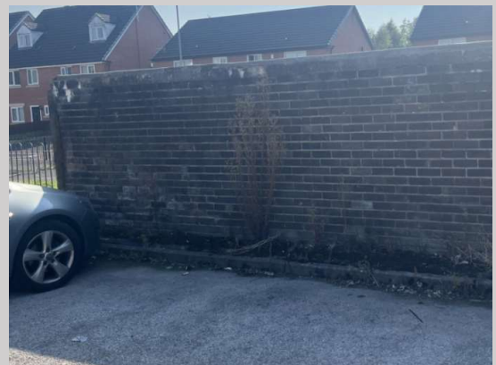
Photograph 6: Sealed back external wall, facing into community car park.
