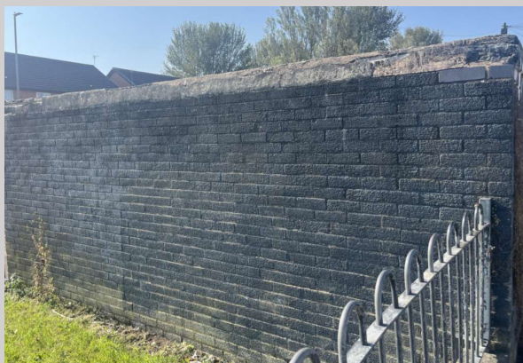
Photograph 5: Sealed side wall with no gaps or crevices.
