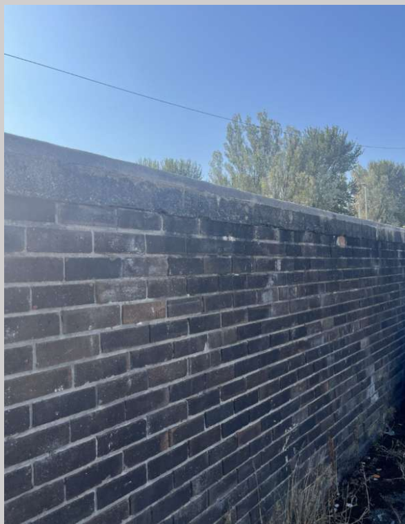
Photograph 9: Back external wall facing car park.
