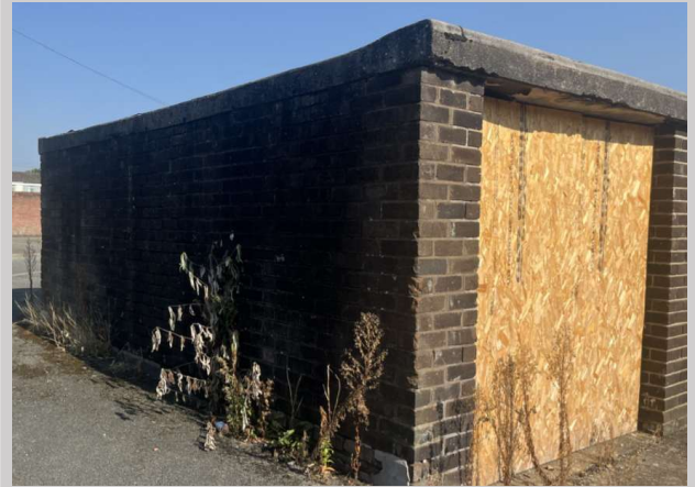
Photograph 8: Fully sealed corner and garage opening.
