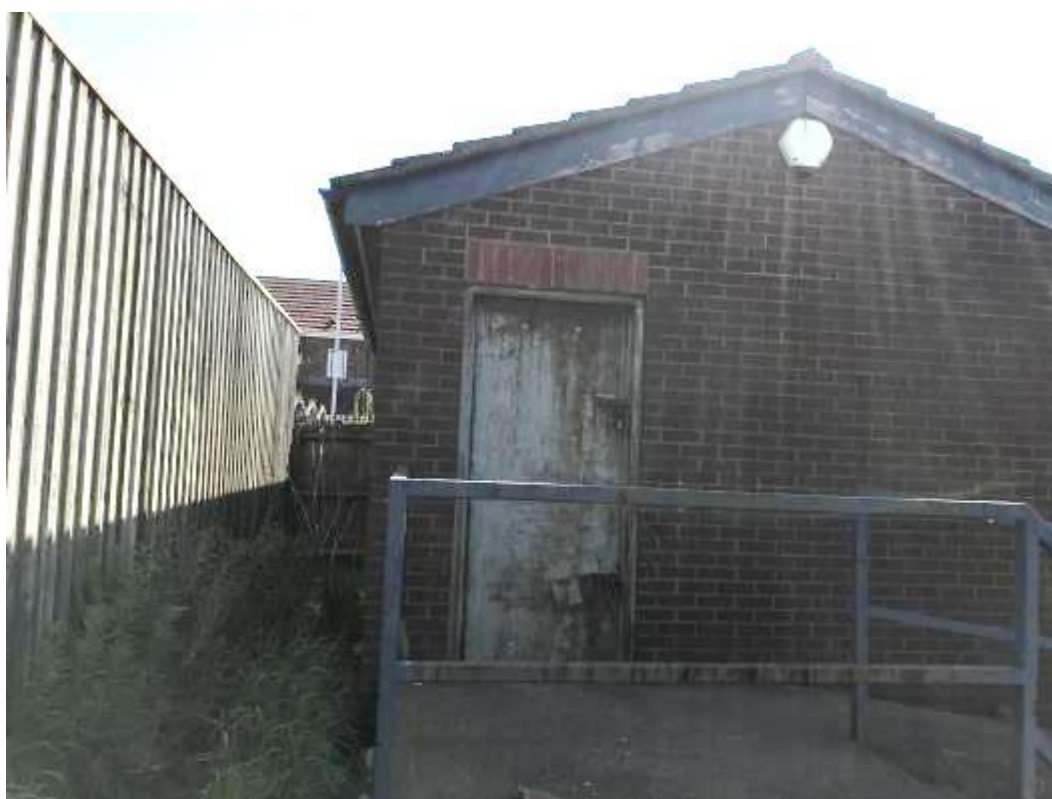
Plate 4 – Viewed from the west
