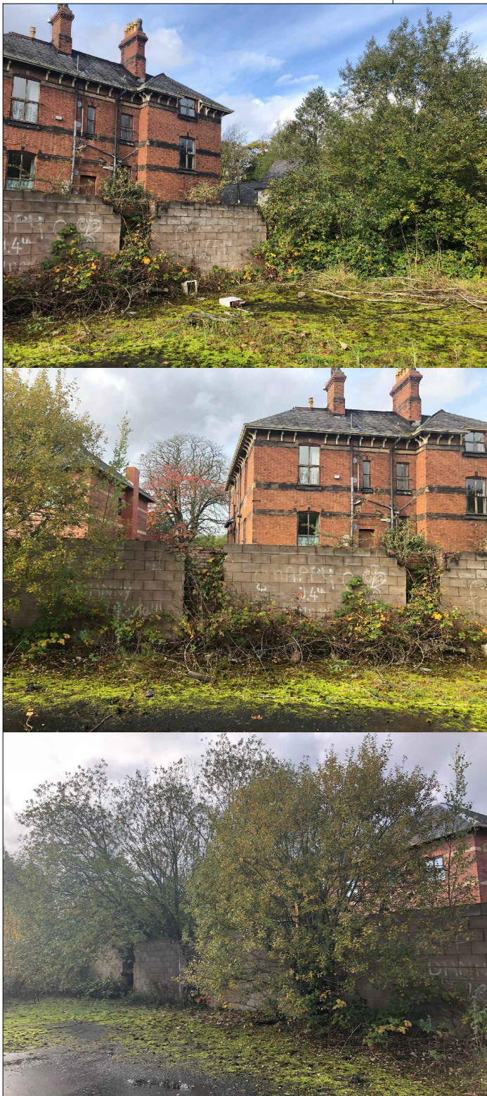
Existing Boundary Wall Photos (Wall to be replaced as detail below)
