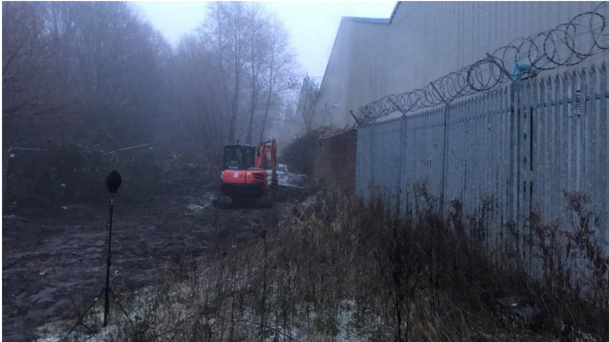
Figure 3: Picture Showing Monitoring Position 1
