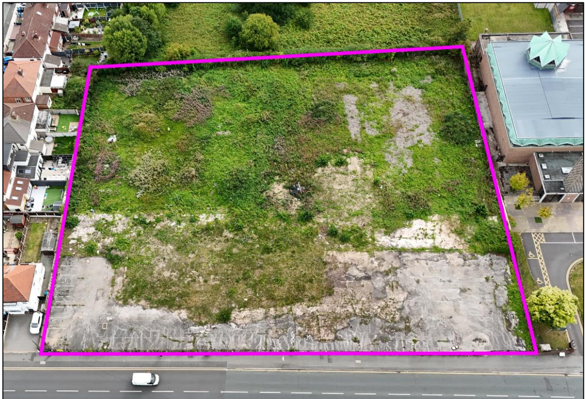
Figure 1: Drone image of the site dated August 2025, looking south to north. The site boundary is highlighted in pink.
