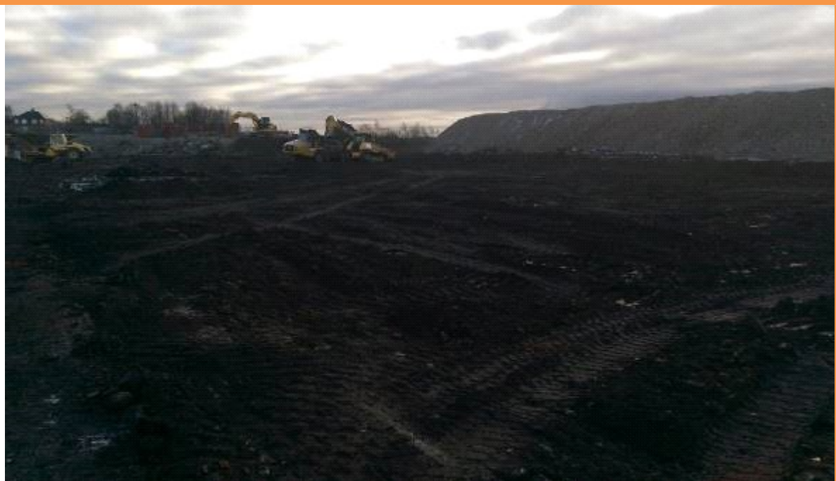
PLATE 10 – REMEDIATION AND TURNOVER COMPLETE IN UPPER AREA OF PARCEL C
