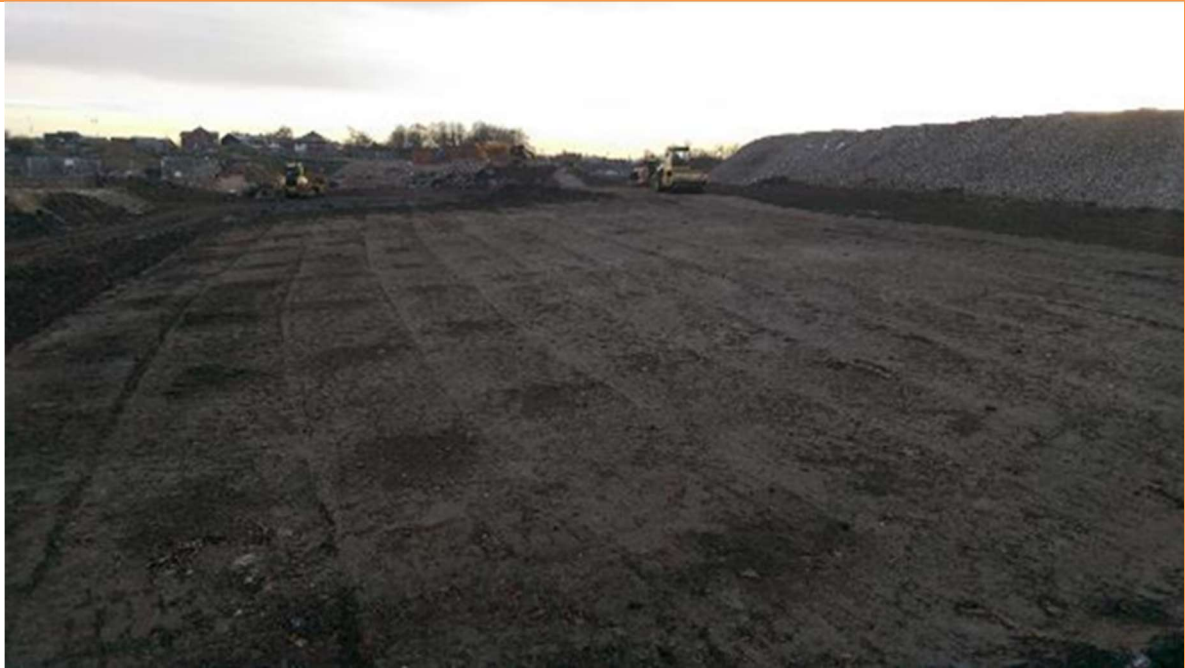
PLATE 13 – VIEW EAST FROM PARCEL C REMEDIATION COMPLETE
