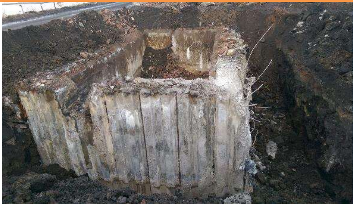
PLATE 7 – REMOVAL OF CONCRETE BELOW GROUND STORAGE TANK
