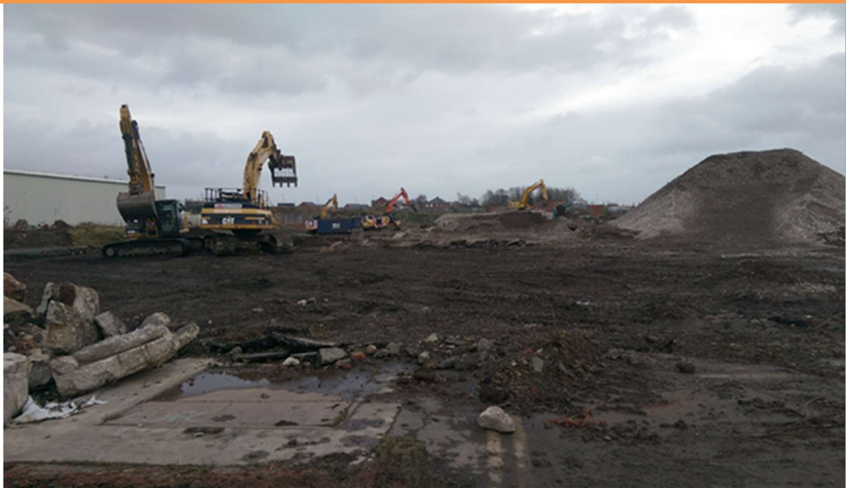
PLATE 3 –PRE-REMEDIATION LOOKING EAST FROM CENTER OF PARCEL C
