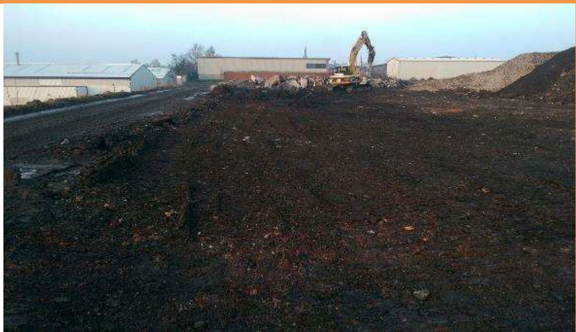
PLATE 12 – REMEDIATED SOILS BEING RE-GRADED TO FORMATION LEVELS
