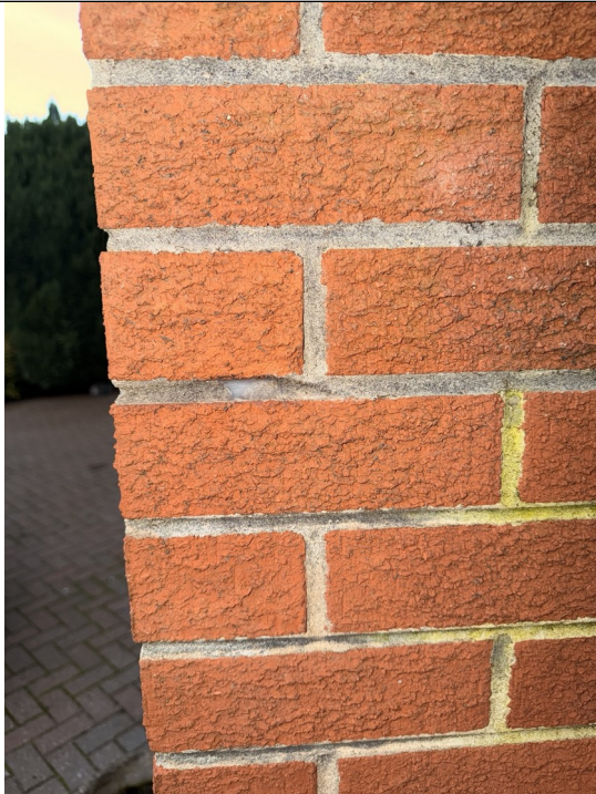
Existing brick face texture and grey mortar joints.
