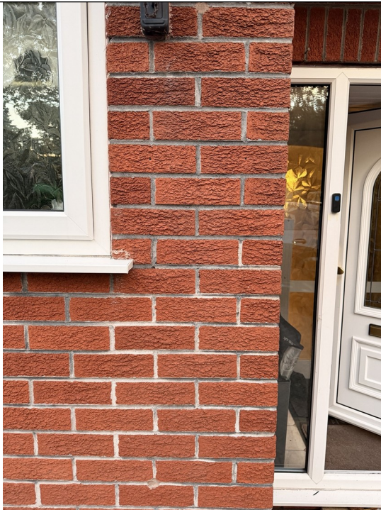
Existing brickwork reference - principal wall close-up.
