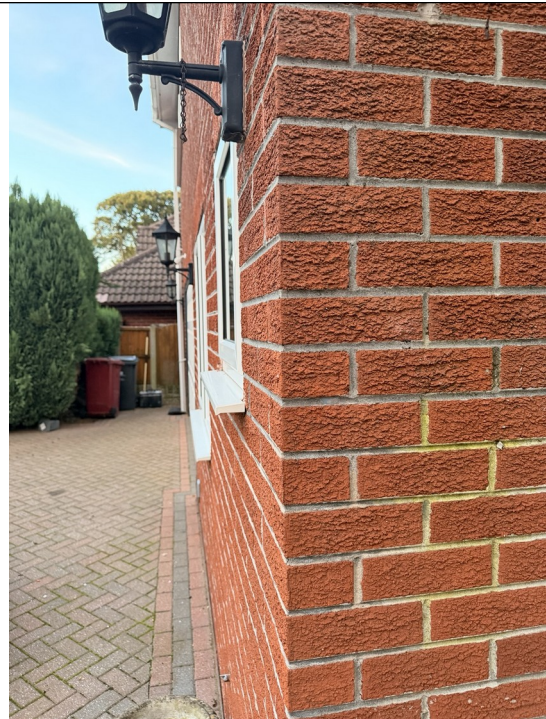
Existing brickwork reference - corner and wider context.
