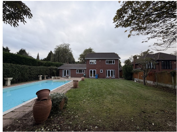
Figure 3. Existing rear elevation and wider rear-garden context.
