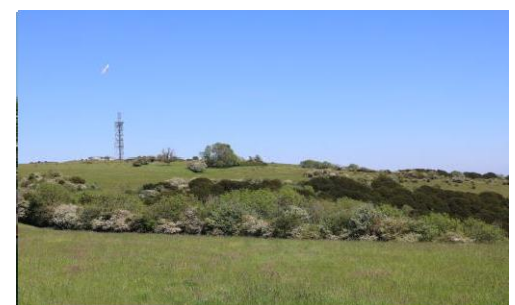
South Downs National Park 10 number Telecommunications Masts
