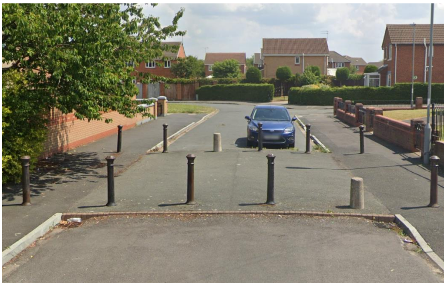
Figure 2-5 - Bollards on Roseheath Drive
