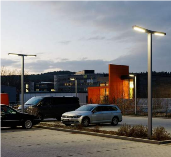
Utilising multi-head lighting columns for car park
