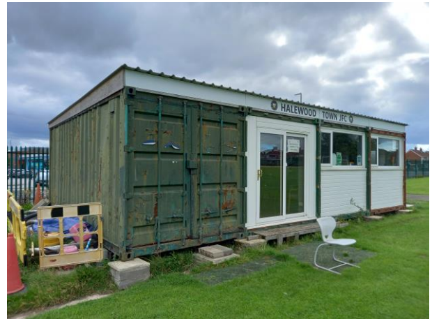
Photograph 20 – Metal storage container (B5) modified with cladding, roofing sheet, UPVC windows and door. Adjacent to B4. Low PBRA.
