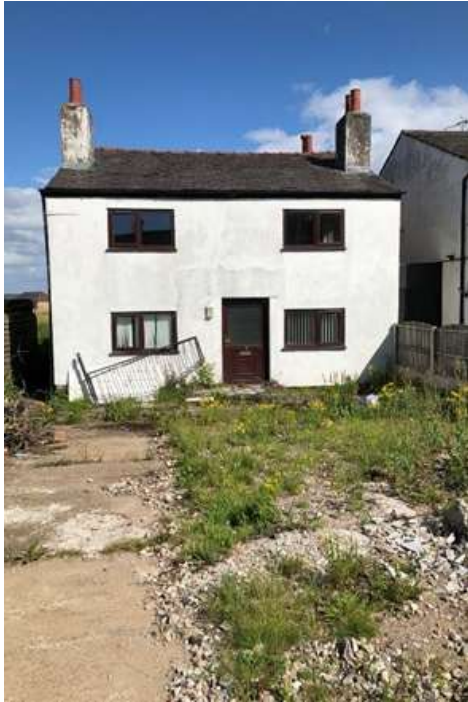
Photo 1: General view of Building 1 from Bailey's Lane (west)
