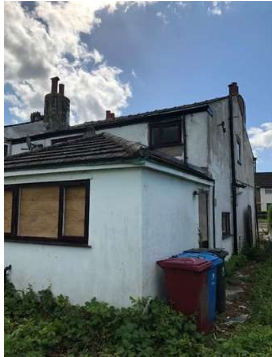
Photo 2: General view of Building 1 – eastern elevation and northern gable end
