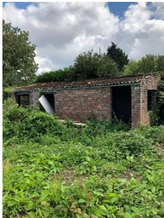
Photo 4: General view of Building 2.
