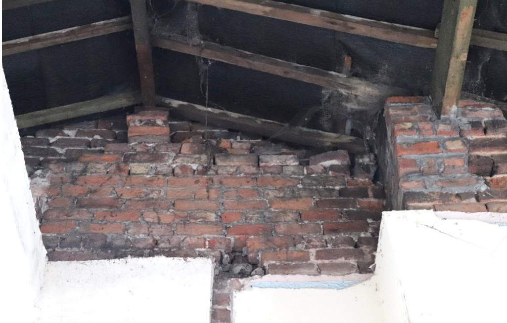
Figure 3: External Wall Brickwork, from room C
