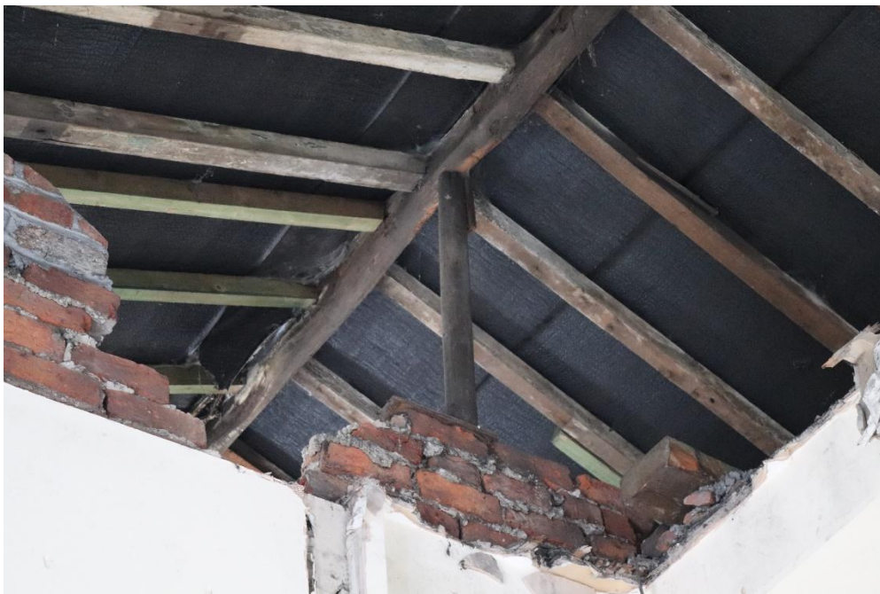
Figure 6: Roof timber, viewed from Room B
