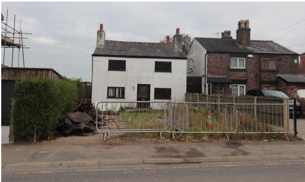
Figure 2: Photograph of 75 Baileys Lane (white dwelling in centre of image)
