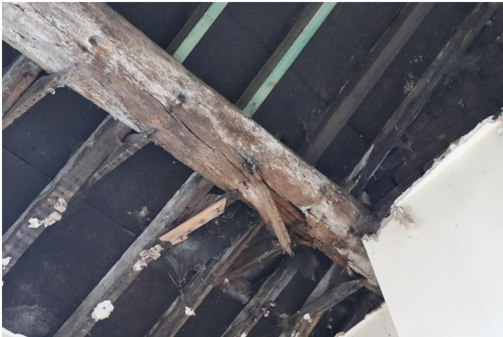
Figure 5: Principal purlin on rear pitch, Room C
