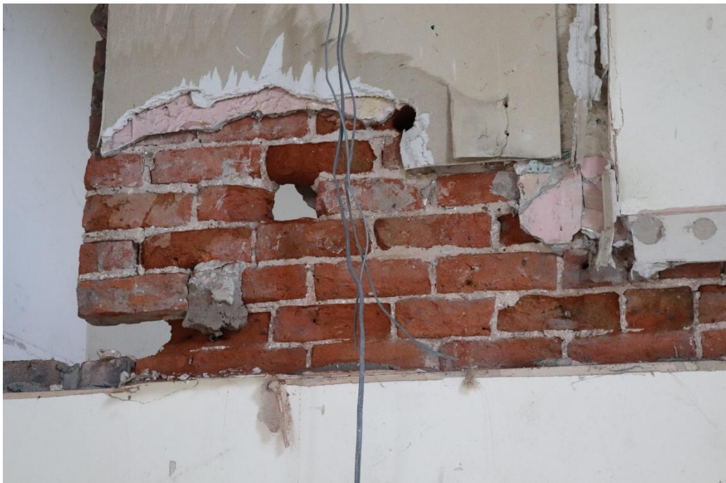
Figure 4: Internal Wall Brickwork, from Room C
