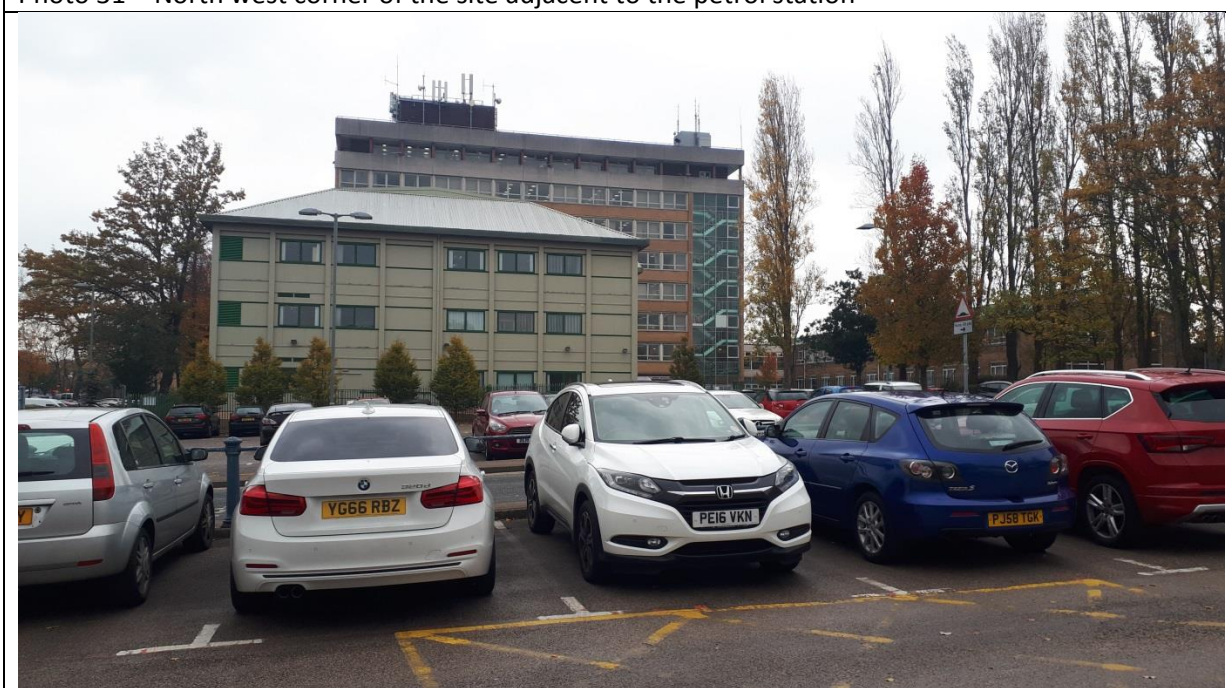
Photo 32 – Car park to the centre of the site
