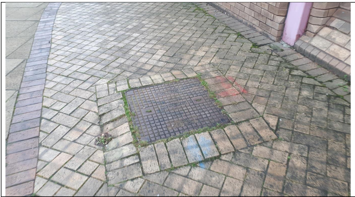
Photo 11 – Evidence of services on site
