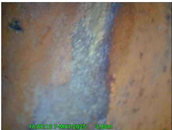
3, 00:00:32, 3.86 m Finish node, other special chamber, reference: Downpipe, Internal downpipe reached
