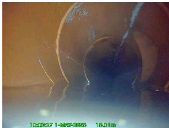
6, 00:01:32, 15.01 m Junction at 3 o'clock, 150mm dia
