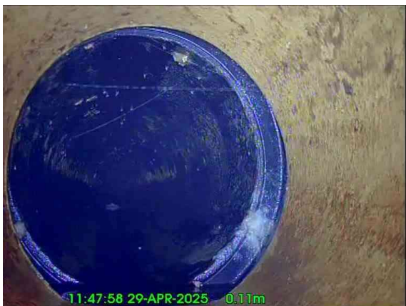
1, 00:00:06, 0.11 m Pipe material changes to pitch fibre at this point
