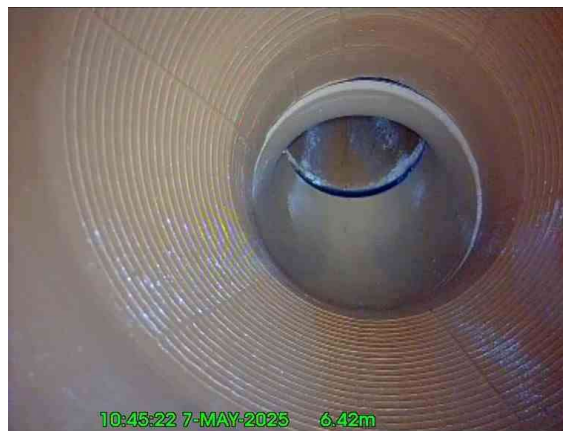
4, 00:00:33, 6.42 m Pipe size changes, new size(s), 150mm high
