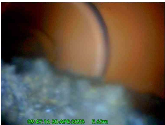
3, 00:02:18, 5.63 m Line deviates left
