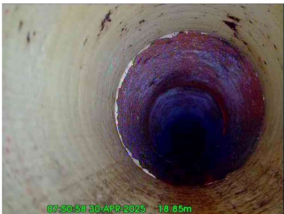
5, 00:00:59, 18.85 m Point repair, localised lining from 12 o'clock to 12 o'clock, finish
