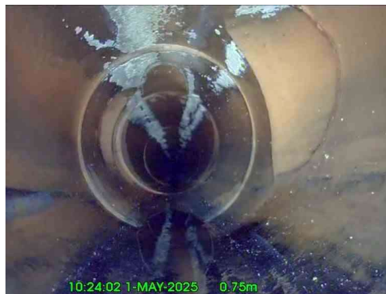
2, 00:00:07, 0.75 m Junction at 2 o'clock, 150mm dia
