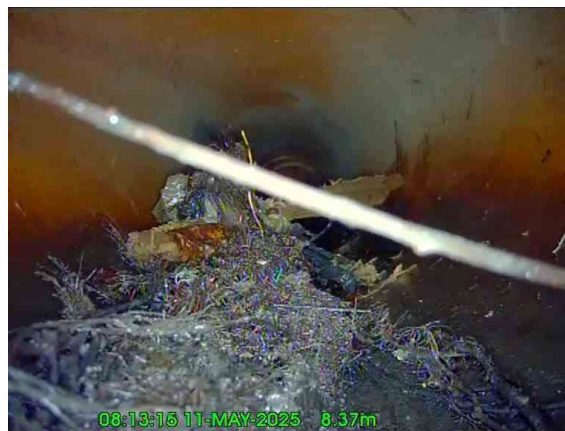
4, 00:01:41, 8.37 m Roots, mass, 25% cross-sectional area loss
