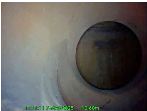
7, 00:00:56, 10.80 m Junction at 6 o'clock, 225mm dia, External Backdrop
