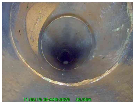
6, 00:01:54, 32.55 m Junction at 10 o'clock, 150mm dia
