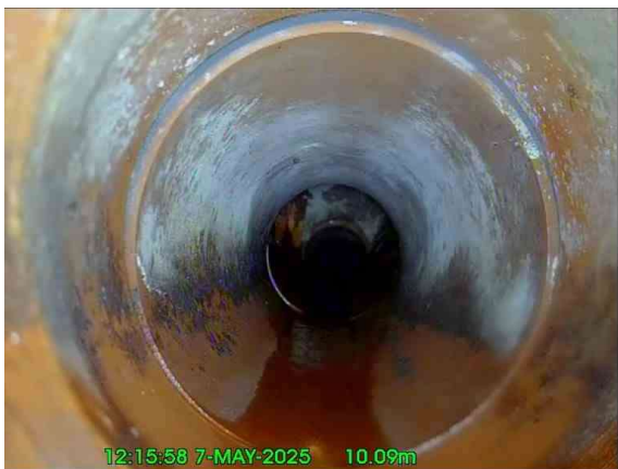
3, 00:00:40, 10.09 m Pipe size changes, new size(s), 150mm high
