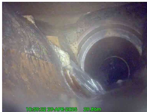
6, 00:02:15, 29.86 m Finish node, manhole, reference: MH outside of survey site boundary reached, UU MH Ref: 2901
