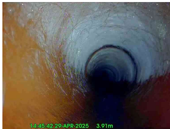
2, 00:00:27, 3.91 m Roots, mass, 20% cross-sectional area loss, finish
