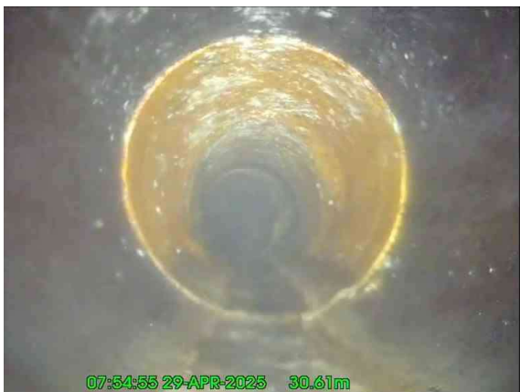
9, 00:02:30, 30.61 m Pipe material changes to vitrified clay at this point
