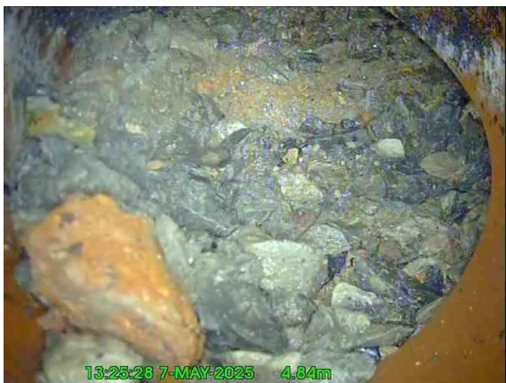
3, 00:00:33, 4.84 m Finish node, other special chamber, reference: Capped, Capped pipe reached
