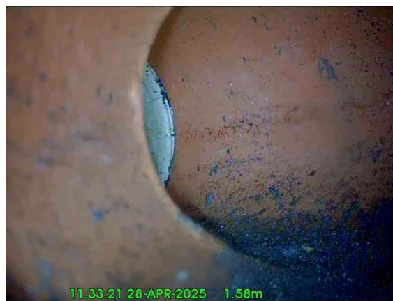
4, 00:00:28, 1.58 m Finish node, major connection without manhole, reference: Main sewer between MH2 UTL and MH5 reached
