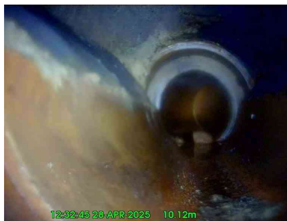
4, 00:01:25, 10.12 m Finish node, manhole, reference: MH6 UTL (Buried MH) reached
