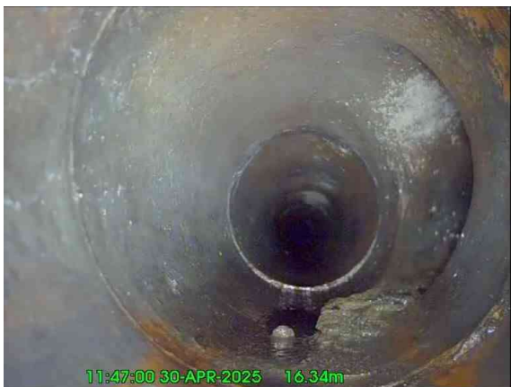
3, 00:01:05, 16.34 m Junction at 3 o'clock, 150mm dia
