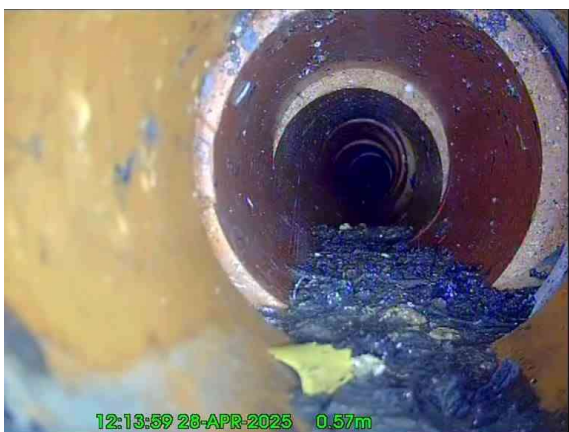
3, 00:00:14, 0.57 m Pipe material changes to vitrified clay at this point
