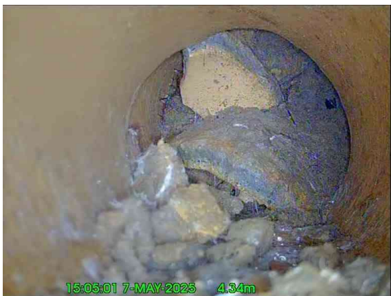
3, 00:00:24, 4.34 m Finish node, other special chamber, reference: Capped, Capped pipe reached
