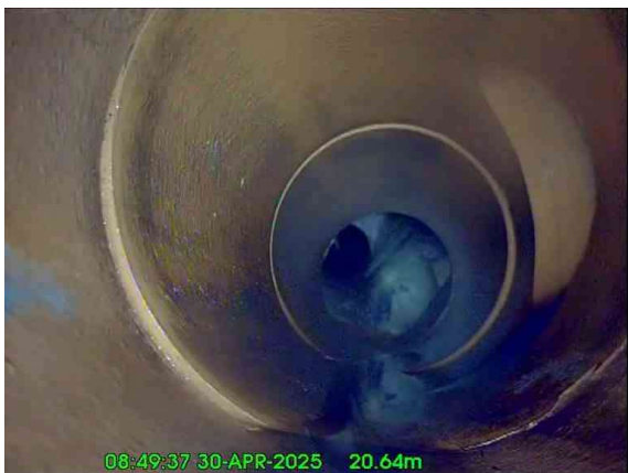
5, 00:01:33, 20.64 m Junction at 2 o'clock, 150mm dia
