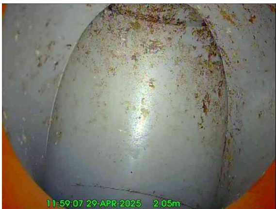
3, 00:00:20, 2.05 m Finish node, manhole, reference: MH30 reached, Internal Backdrop visible
