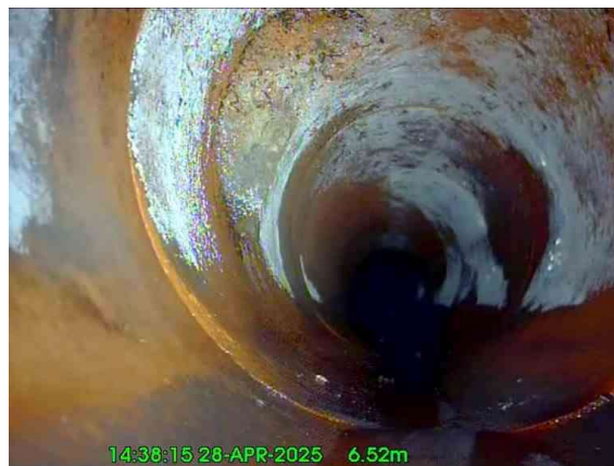
2, 00:00:41, 6.52 m Junction at 10 o'clock, 100mm dia
