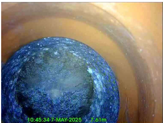
7, 00:00:45, 7.61 m Finish node, rodding eye, reference: RE reached
