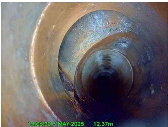
5, 00:00:46, 12.37 m Junction at 10 o'clock, 150mm dia, from Gully3 X
