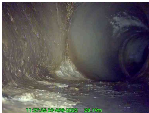
14, 00:01:53, 28.19 m Finish node, manhole, reference: MH outside of survey site boundary reached, UU MH Ref: 2903
