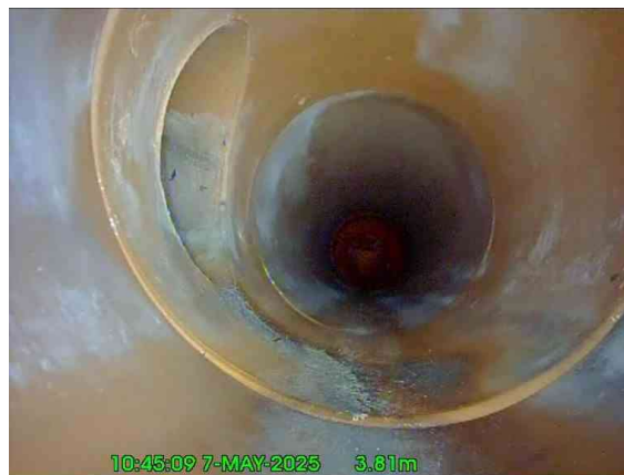
2, 00:00:20, 3.81 m Junction at 9 o'clock, 150mm dia, from Gully2 X
