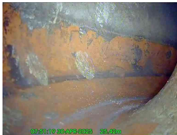
8, 00:01:21, 25.42 m Finish node, manhole, reference: MH at exit to ASDA petrol station site reached
