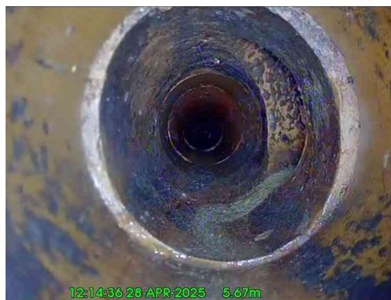
8, 00:00:51, 5.67 m Junction at 3 o'clock, 100mm dia
