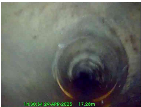
3, 00:01:09, 17.28 m Junction at 3 o'clock, 150mm dia
