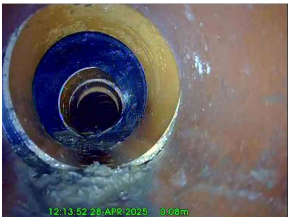
1, 00:00:02, 0.08 m Pipe material changes to polyvinyl chloride at this point
