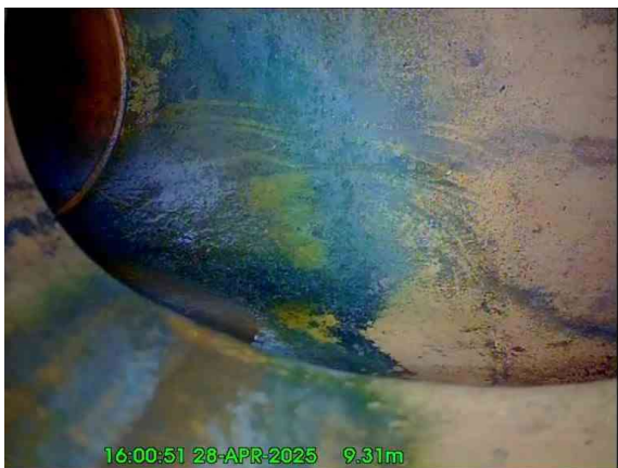
7, 00:00:59, 9.31 m Finish node, major connection without manhole, reference: Main public sewer between MH15 and MH23 reached
