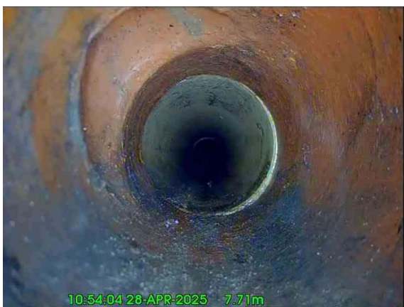
3, 00:00:44, 7.71 m Junction at 10 o'clock, 100mm dia
