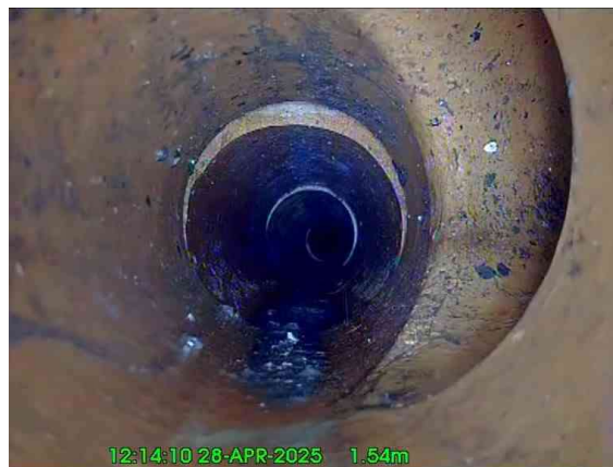
6, 00:00:25, 1.54 m Junction at 3 o'clock, 100mm dia
