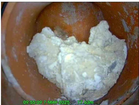
7, 00:01:48, 17.63 m Finish node, other special chamber, reference: Downpipe, Internal downpipe reached
