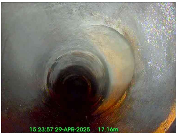
3, 00:01:31, 17.16 m Junction at 3 o'clock, 150mm dia
