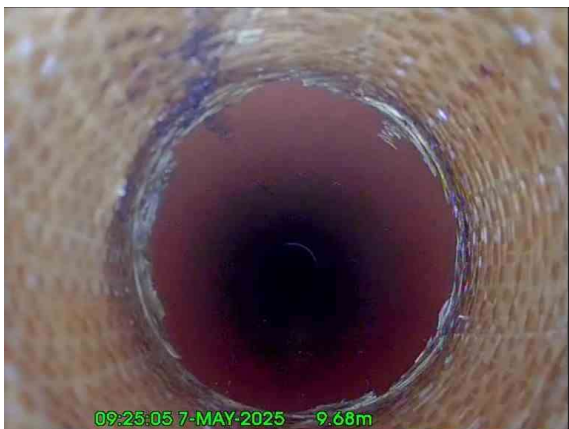
5, 00:00:41, 9.68 m Point repair, localised lining from 12 o'clock to 12 o'clock, finish
