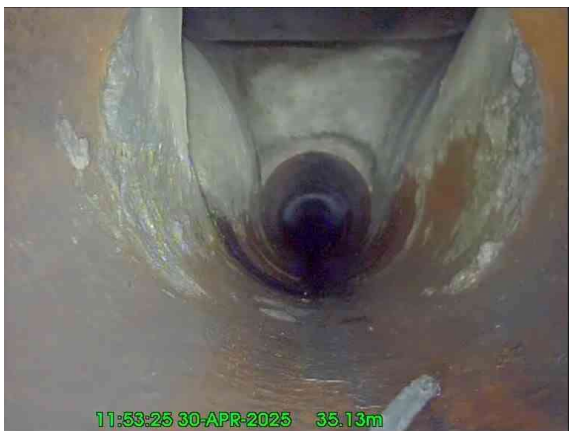
7, 00:03:03, 35.13 m Finish node, manhole, reference: MH at entrance to ASDA petrol station site reached
