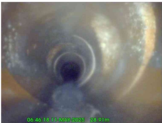
7, 00:02:06, 28.91 m Junction at 2 o'clock, 150mm dia
