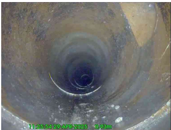
3, 00:00:11, 0.93 m Junction at 2 o'clock, 100mm dia
