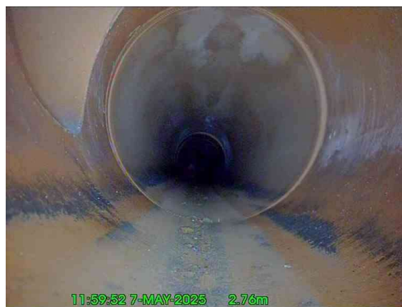
2, 00:00:17, 2.76 m Junction at 10 o'clock, 150mm dia
