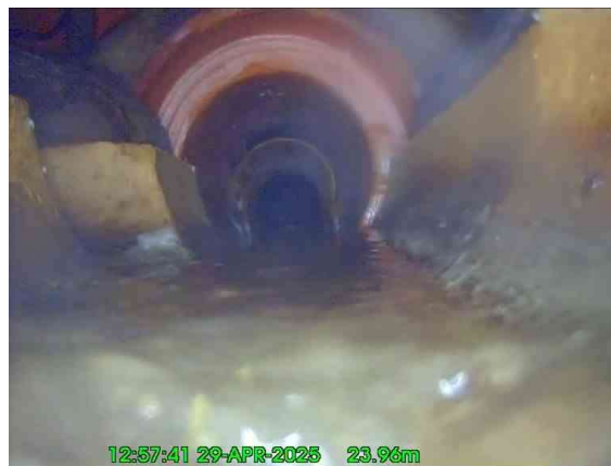
10, 00:01:32, 23.96 m Finish node, manhole, reference: MH20 UTL (Buried MH) reached
