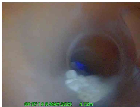
4, 00:00:23, 4.72 m Junction at 2 o'clock, 100mm dia
