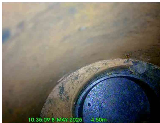
4, 00:00:29, 4.50 m Finish node, gully, reference: Buried Gly reached
