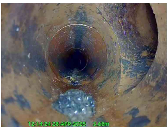
7, 00:00:39, 3.65 m Junction at 3 o'clock, 100mm dia
