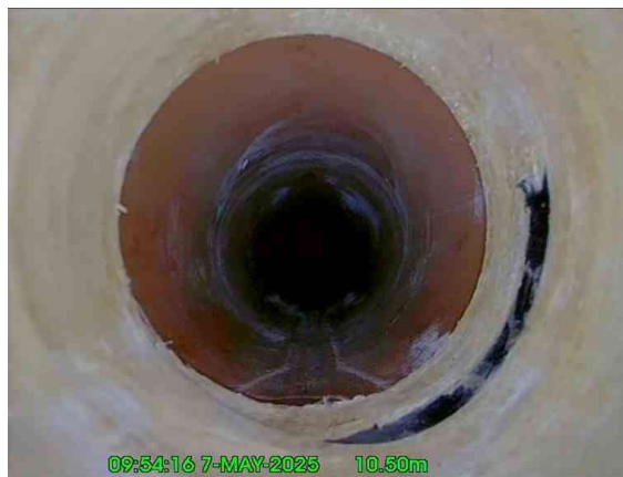
4, 00:00:56, 10.50 m Point repair, localised lining from 12 o'clock to 12 o'clock, finish
