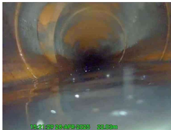
6, 00:03:20, 22.03 m Junction at 10 o'clock, 100mm dia, from MH18 X
