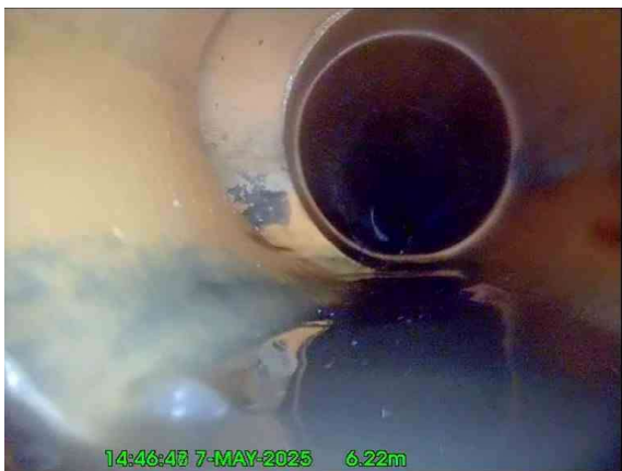
3, 00:00:41, 6.22 m Junction at 9 o'clock, 150mm dia
