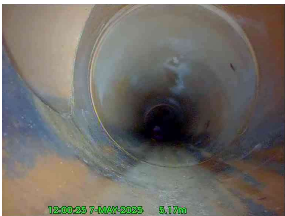
3, 00:00:50, 5.17 m Junction at 10 o'clock, 150mm dia
