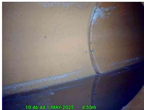
6, 00:00:43, 4.55 m Finish node, major connection without manhole, reference: Main public sewer between MH13 and MH10 reached
