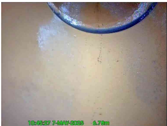
5, 00:00:38, 6.78 m Line deviates up
