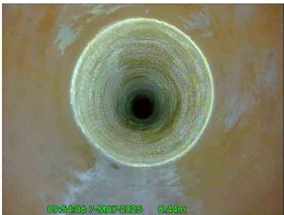
3, 00:00:46, 8.44 m Point repair, localised lining from 12 o'clock to 12 o'clock, start
