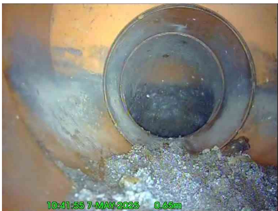
3, 00:00:10, 0.65 m Pipe size changes, new size(s), 150mm high
