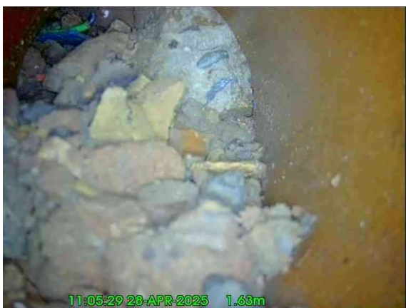
3, 00:00:22, 1.63 m Finish node, other special chamber, reference: Capped, Capped pipe reached
