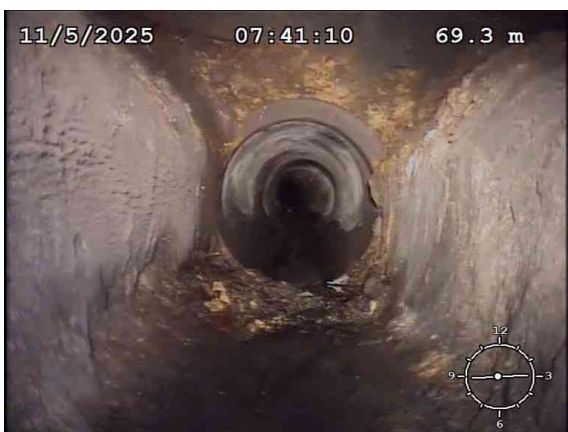
15, 00:07:27, 69.30 m Finish node, manhole, reference: MH67 UTL reached, UU MH Ref: 0802
