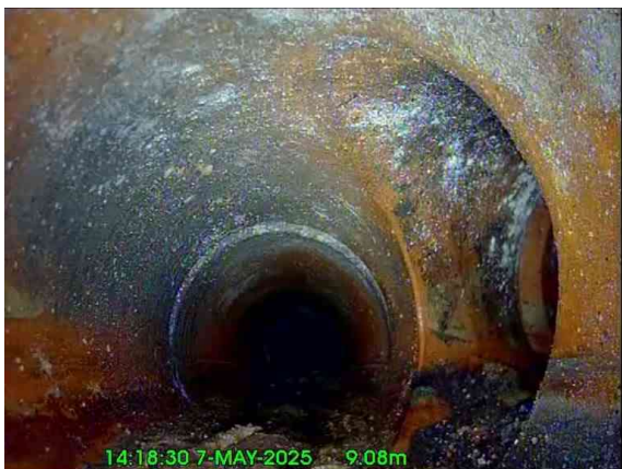
5, 00:00:44, 9.08 m Junction at 3 o'clock, 150mm dia
