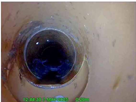
1, 00:00:08, 0.20 m Junction at 6 o'clock, 100mm dia, External Backdrop
