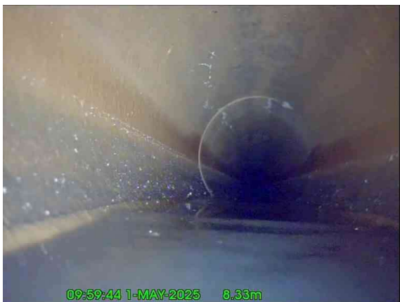
5, 00:00:49, 8.33 m Water level, 10% of the vertical dimension
