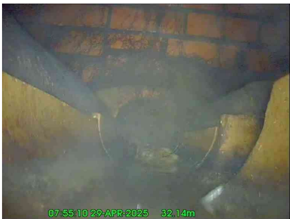
11, 00:02:45, 32.14 m Finish node, manhole, reference: MH20 UTL (Buried MH) reached
