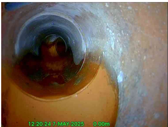
1, 00:00:02, 0.00 m Junction at 6 o'clock, 100mm dia, External Backdrop
