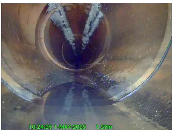
3, 00:00:11, 1.25 m Junction at 10 o'clock, 150mm dia
