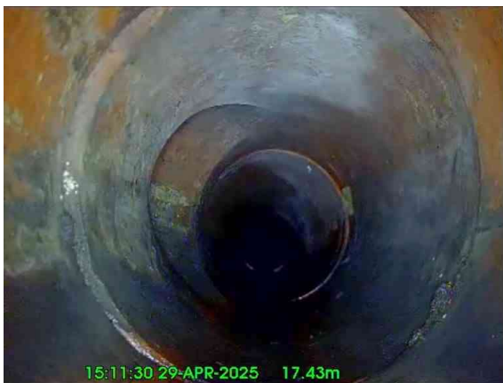
3, 00:01:14, 17.43 m Junction at 10 o'clock, 150mm dia
