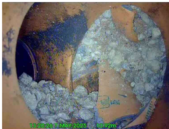
4, 00:00:44, 10.92 m Junction at 9 o'clock, 100mm dia
