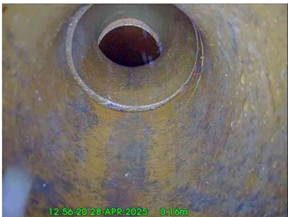
1, 00:00:05, 0.16 m Line deviates up
