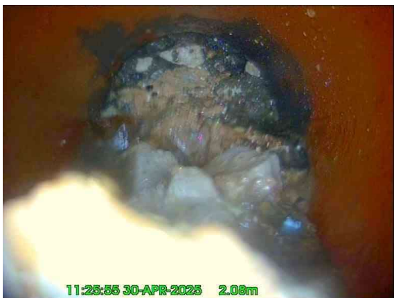
3, 00:00:23, 2.08 m Finish node, other special chamber, reference: Capped, Capped pipe reached
