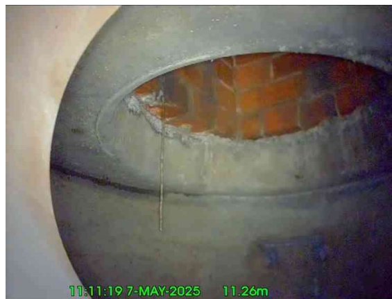
8, 00:01:04, 11.26 m Finish node, manhole, reference: MH53 reached
