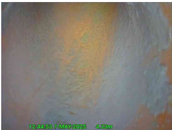
3, 00:00:32, 4.33 m Finish node, other special chamber, reference: Downpipe, Internal downpipe reached
