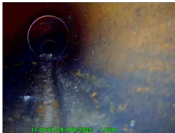
2, 00:00:21, 1.02 m Line deviates up
