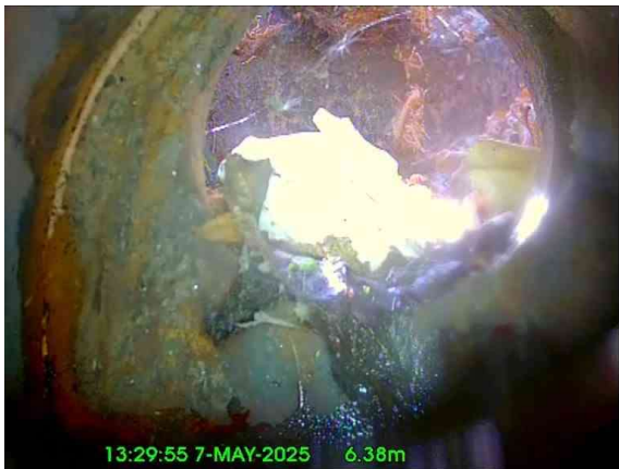
3, 00:00:53, 6.38 m Finish node, gully, reference: Gully reached
