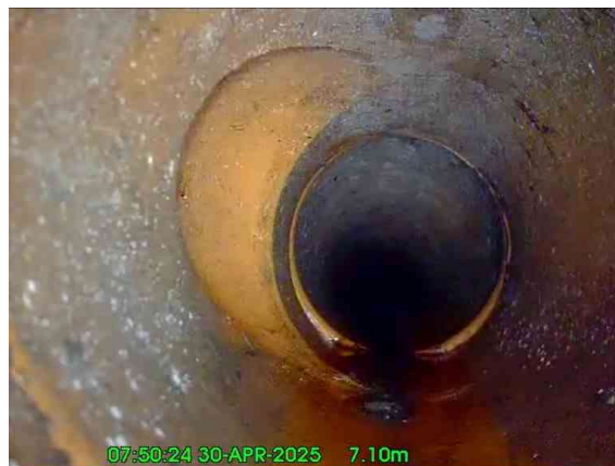
2, 00:00:25, 7.10 m Junction at 9 o'clock, 150mm dia
