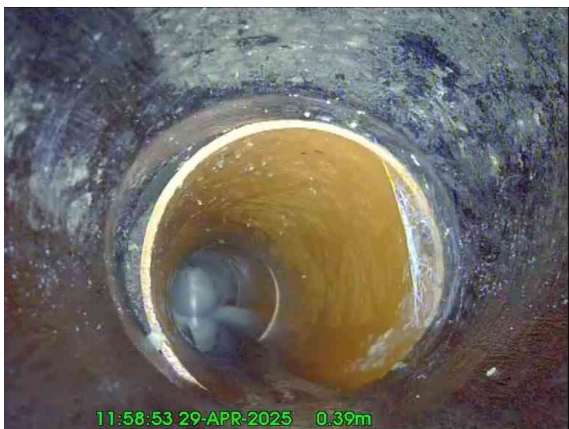
1, 00:00:06, 0.39 m Pipe material changes to polyvinyl chloride at this point
