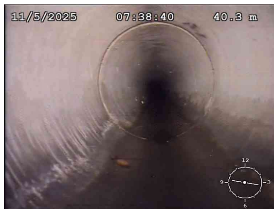
10, 00:04:57, 40.30 m General photograph taken at this point
