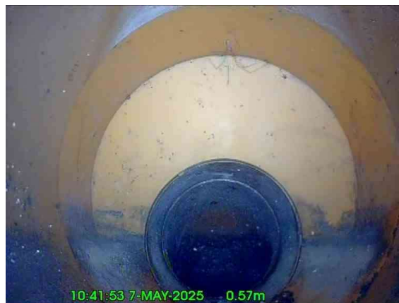
2, 00:00:08, 0.57 m Pipe material changes to polyvinyl chloride at this point
