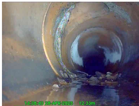
4, 00:01:09, 12.33 m Junction at 11 o'clock, 100mm dia
