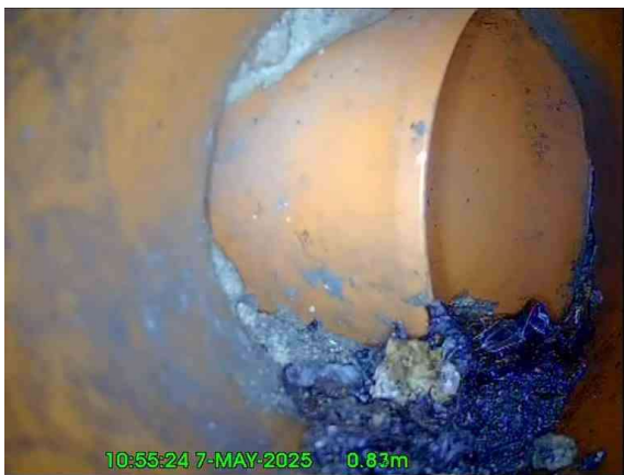
3, 00:00:17, 0.83 m Finish node, other special chamber, reference: Vent Pipe, Vent Pipe reached
