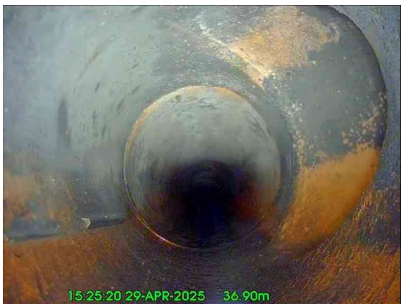
7, 00:02:54, 36.90 m Junction at 2 o'clock, 150mm dia
