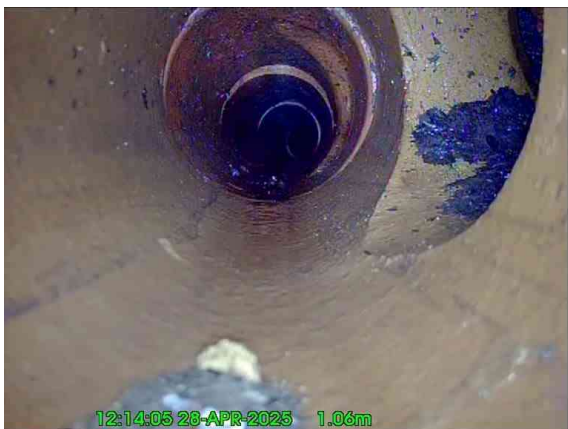
5, 00:00:20, 1.06 m Junction at 3 o'clock, 100mm dia
