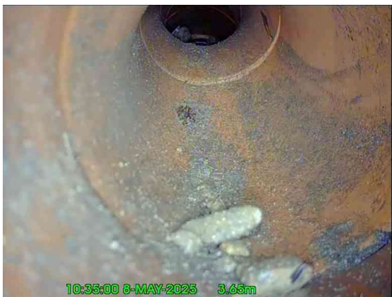
3, 00:00:21, 3.65 m Line deviates up
