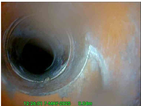
1, 00:00:08, 0.04 m Junction at 6 o'clock, 100mm dia, External Backdrop
