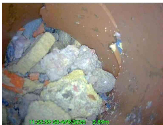
4, 00:00:42, 2.89 m Finish node, other special chamber, reference: Capped, Capped pipe reached
