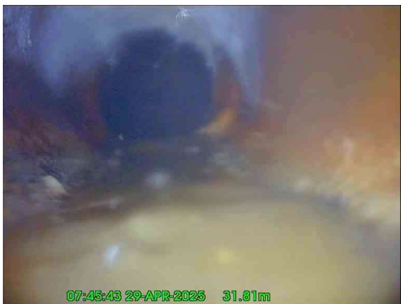
7, 00:01:31, 31.81 m Junction at 6 o'clock, 150mm dia, External Backdrop
