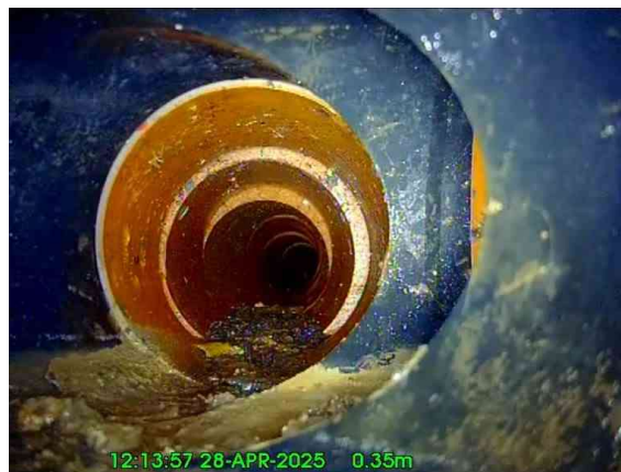
2, 00:00:12, 0.35 m Junction at 3 o'clock, 100mm dia
