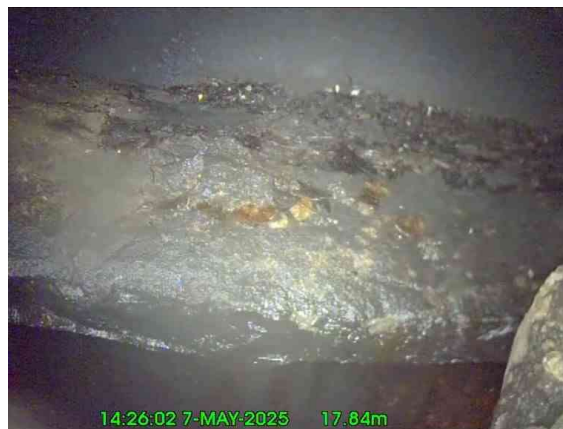
6, 00:00:03, 17.84 m Finish node, manhole, reference: MH outside of survey site boundary reached, UU MH Ref: 2908
