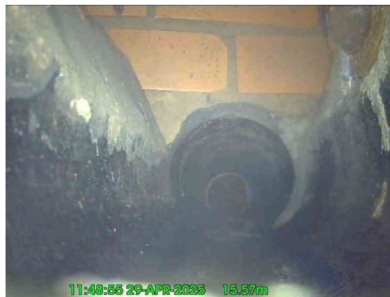
6, 00:01:04, 15.57 m Finish node, manhole, reference: MH29 reached
