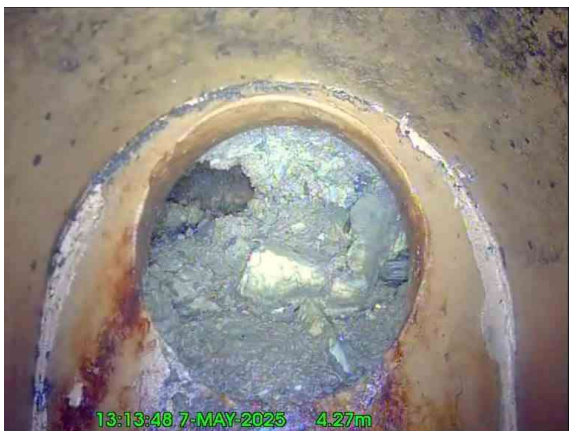
3, 00:00:30, 4.27 m Finish node, gully, reference: Buried Gully reached
