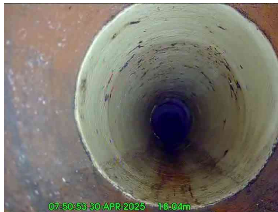
4, 00:00:54, 18.04 m Point repair, localised lining from 12 o'clock to 12 o'clock, start
