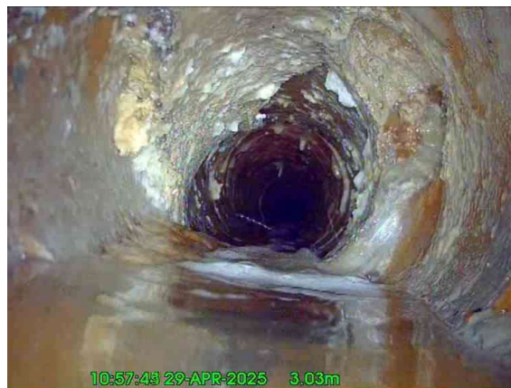
2, 00:00:26, 3.03 m Junction at 2 o'clock, 100mm dia
