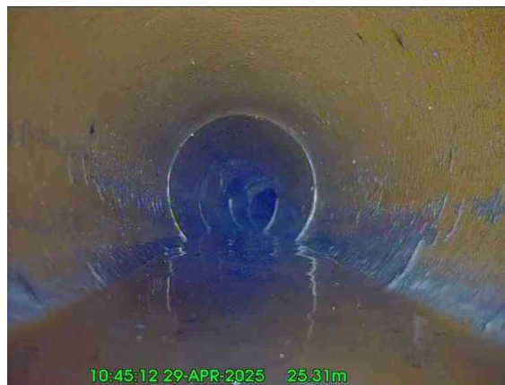
18, 00:02:29, 25.31 m General photograph taken at this point
