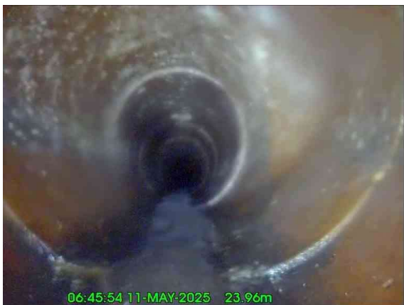
5, 00:01:43, 23.96 m Junction at 3 o'clock, 150mm dia
