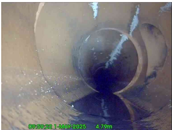
3, 00:00:27, 4.79 m Junction at 3 o'clock, 150mm dia
