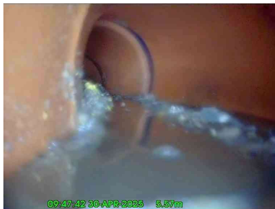
2, 00:02:44, 5.57 m Settled deposits, hard or compacted, 10% cross-sectional area loss, start, Solid set debris remained in sewer following jetting
