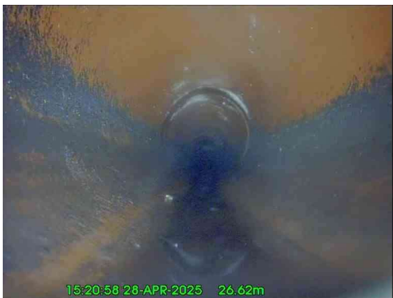
7, 00:02:50, 26.62 m Water level, 5% of the vertical dimension
