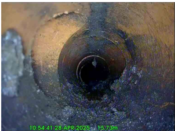
5, 00:01:21, 15.73 m Junction at 10 o'clock, 100mm dia
