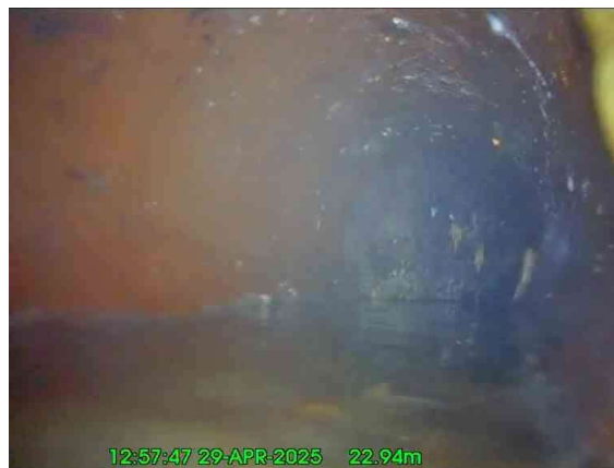
6, 00:01:39, 22.94 m Pipe material changes to vitrified clay at this point
