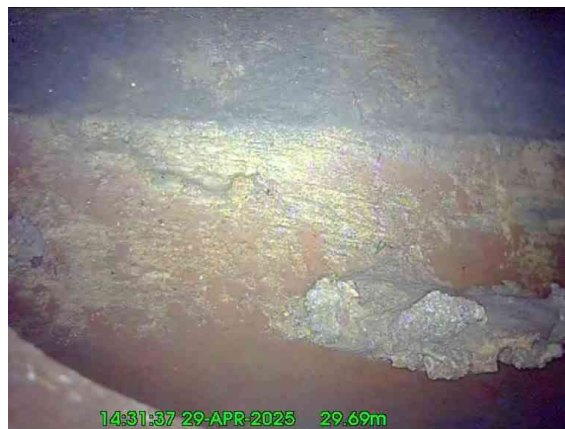
6, 00:01:53, 29.69 m Finish node, manhole, reference: MH at entrance to ASDA petrol station site reached
