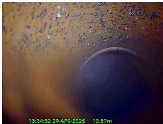
6, 00:01:07, 10.87 m Junction at 6 o'clock, 150mm dia, Internal Backdrop
