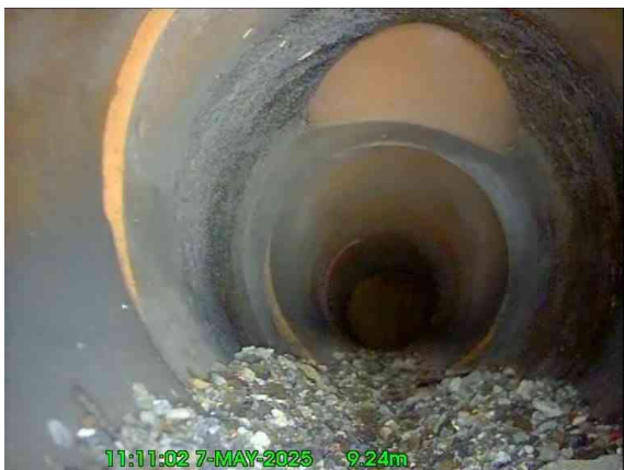
5, 00:00:47, 9.24 m Junction at 12 o'clock, 150mm dia
