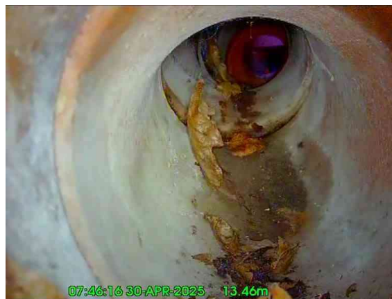
4, 00:01:00, 13.46 m Line deviates up
