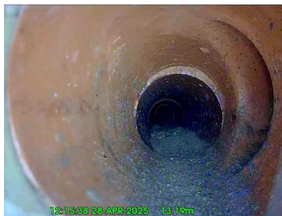
12, 00:01:54, 13.19 m Junction at 3 o'clock, 100mm dia
