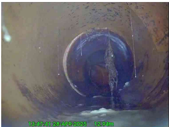
5, 00:01:33, 12.94 m Junction at 2 o'clock, 100mm dia
