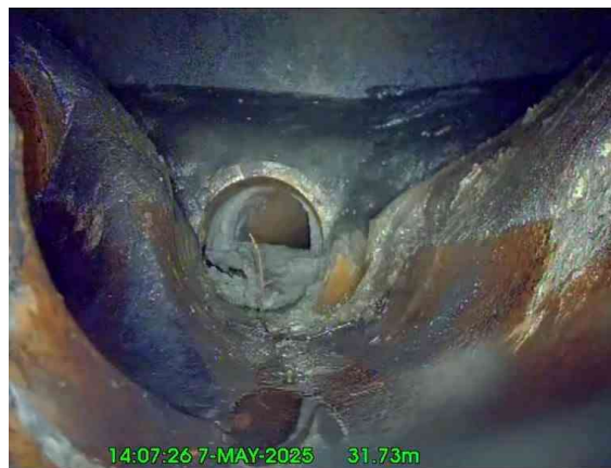
8, 00:01:42, 31.73 m Finish node, manhole, reference: MH60 UTL (MH Under Fence) reached
