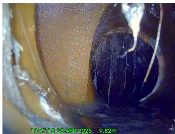
4, 00:01:10, 9.82 m Junction at 9 o'clock, 150mm dia
