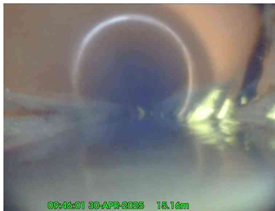
8, 00:01:02, 15.16 m Junction at 2 o'clock, 150mm dia
