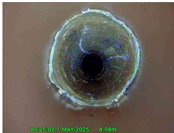
4, 00:00:38, 8.98 m Point repair, localised lining from 12 o'clock to 12 o'clock, start
