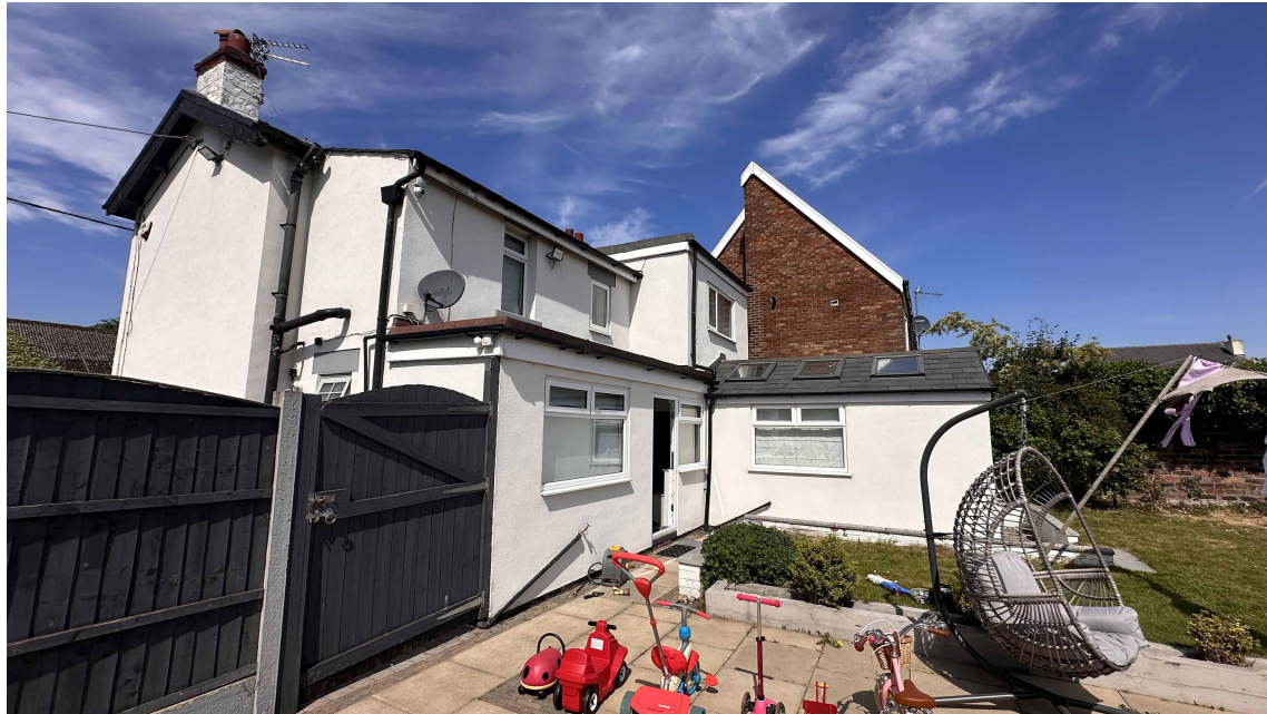
Photo of rear of 15 Chapel Lane towards adjacent property to North
