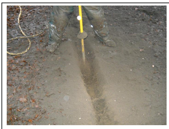
4B: Roots being exposed by compressed air soil displacement excavation using an Air Spade.
